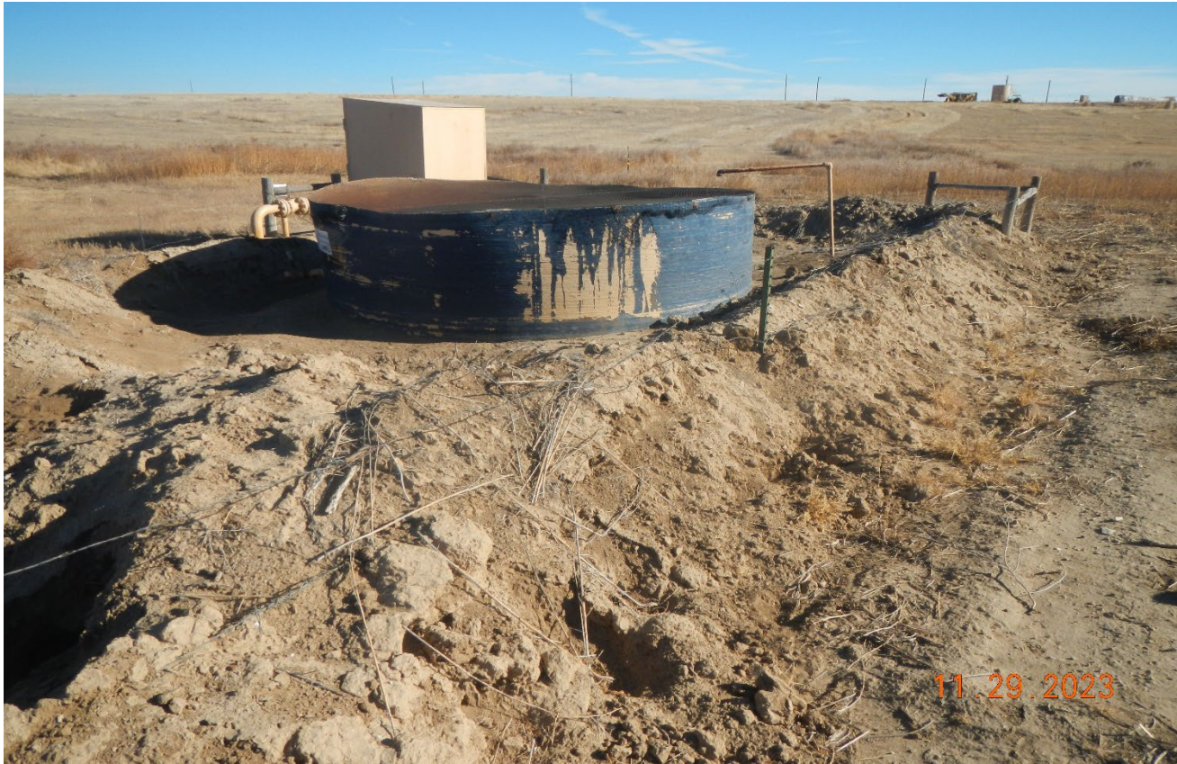
Photo 4. The fence around the open top tank is inadequate to prevent livestock entry and is not maintained. Previous corrective action was not completed.
