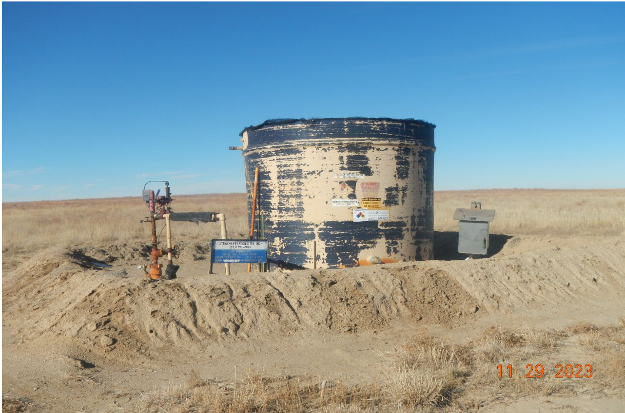
Photo 6. Facing toward the wellsite. The labeling on the tank is faded and peeled off. The berm around the tank has been built up however soils were not compacted to be impermeable.
