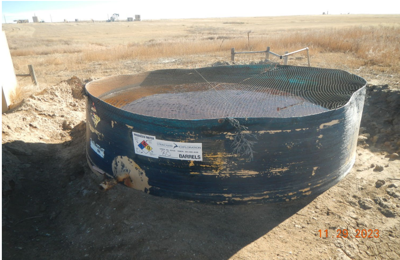
Photo 3. The netting on the open top tank is torn and needs repair. Previous corrective action was not completed.
