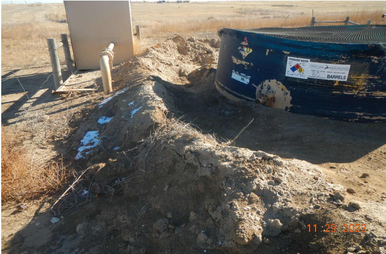
Photo 2. The berm around the tank has been built up however soils were not compacted to be impermeable.
