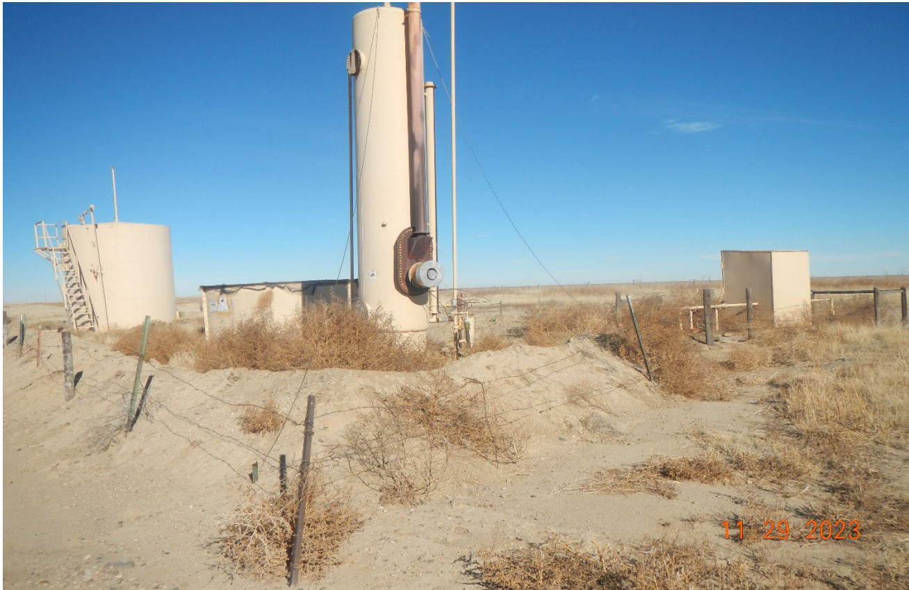
Photo 3. The fence around the tank battery is inadequate to prevent livestock entry and is not maintained. Previous corrective action was not completed.
