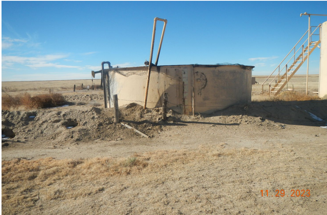
Photo 4. The berm is inadequate to contain a spill as it is piled up against the tank and would spill over the berm along this side. Previous corrective action was not completed.
