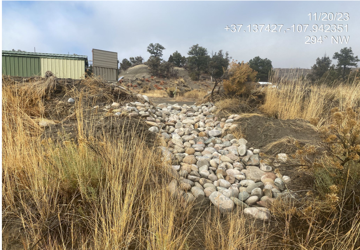
Photo 4. Installed BMPs observed around the location are not per good engineering practice, operator has used round river stone rather than large angular rock. Round rock may increase erosion and scouring in these areas.
