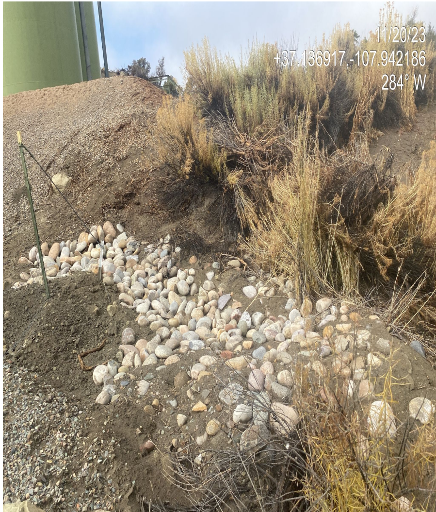
Photo 3. View of stormwater BMPs installed in the eastern interim reclamation area.
