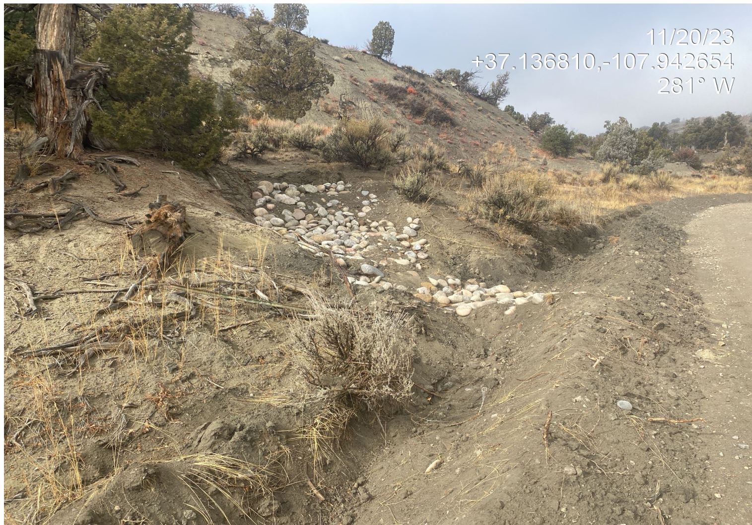
Photo 2. View of stormwater BMPs installed in the western interim reclamation area by the access road.
