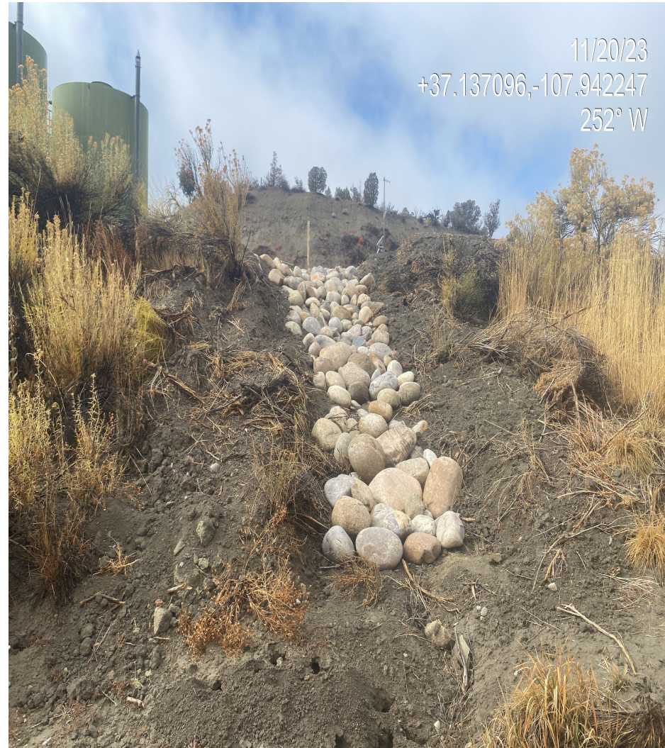
Photo 3. View of stormwater BMPs installed in the eastern interim reclamation area.
