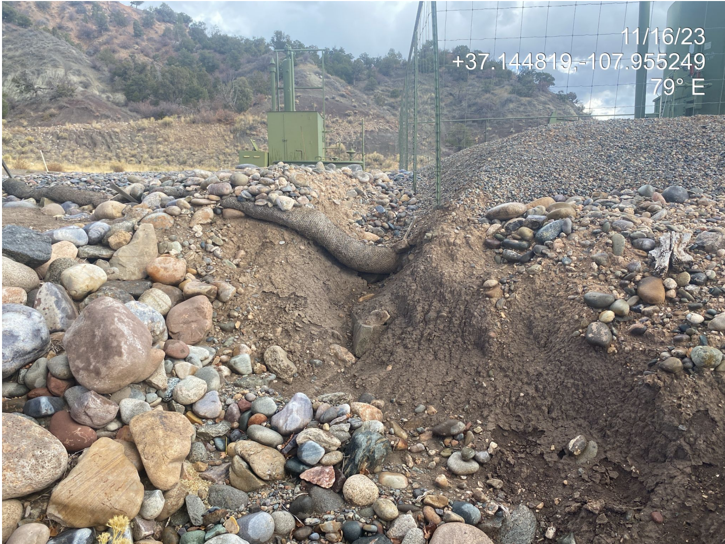
Photo 2. View of failing stormwater BMPs and forming gully erosion observed on the western fill slope/interim area of the disturbance.
