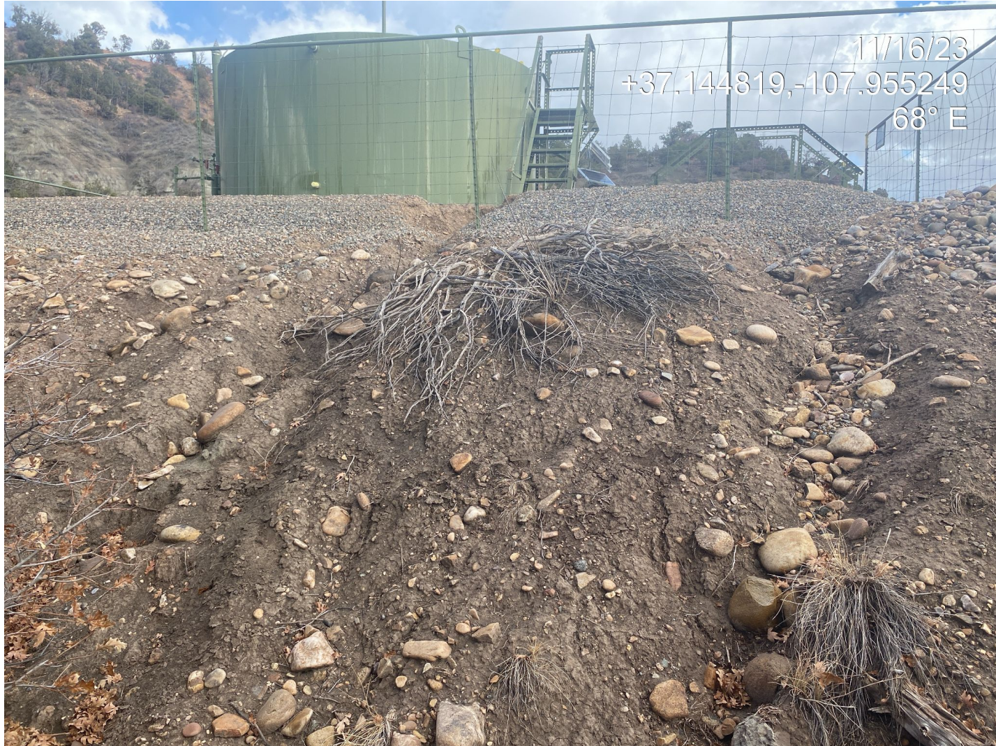
Photo 3. View of additional rill erosion forming on the western fill slope of the disturbance.
