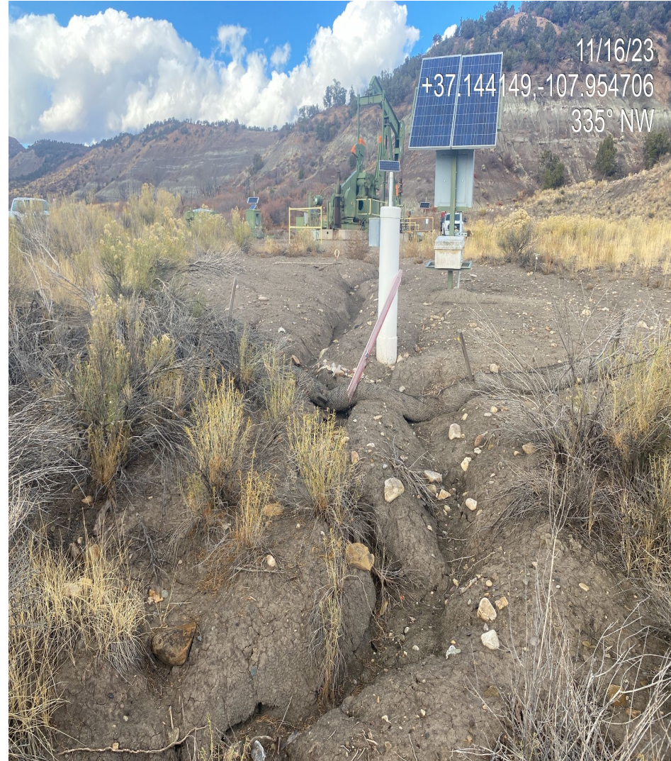
Photo 4. View of rill erosion and failing stormwater BMPs observed in the southern interim area of the disturbance.
