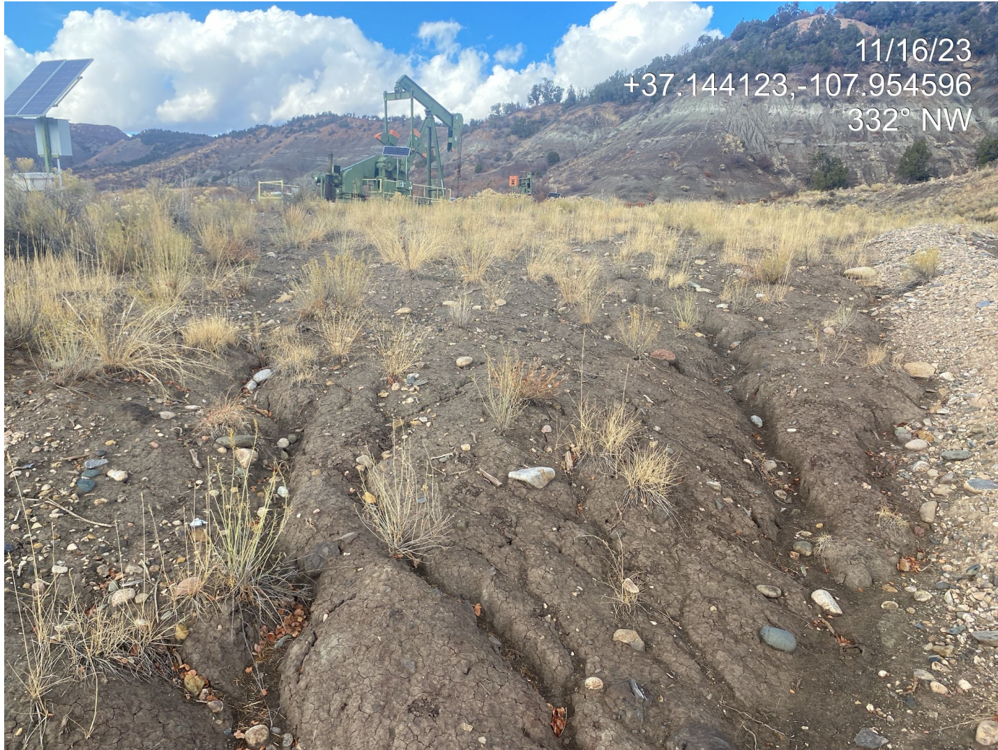
Photo 5. Additional rill erosion forming downslope of failing stormwater BMPs in the southern interim reclamation area.
