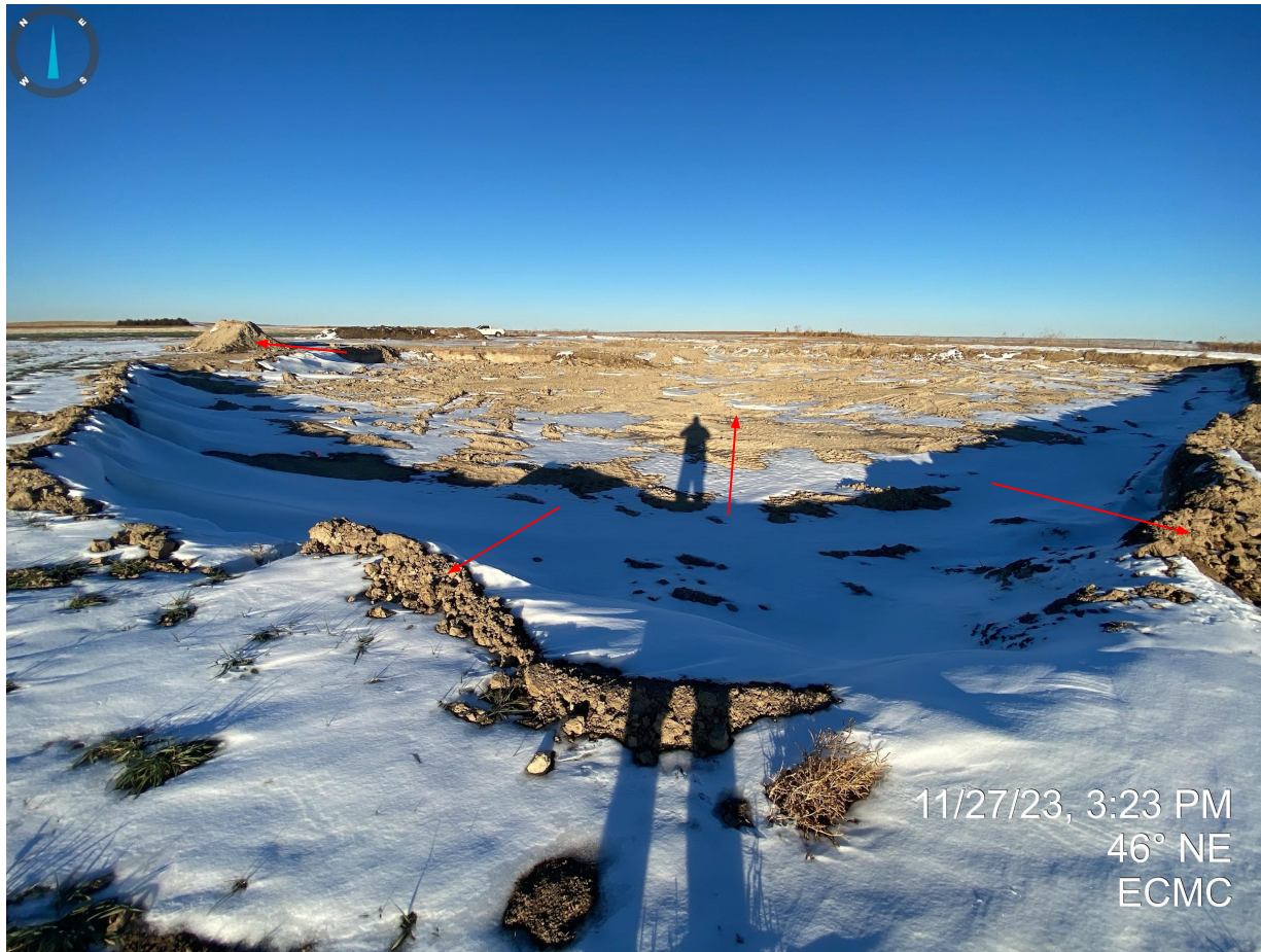
Photo 3. Taken from the southwestern corner of the excavated pit. Stockpiled and exposed soils are not protected from wind and water erosion as they are unconsolidated and not properly stabilized in their current state.
