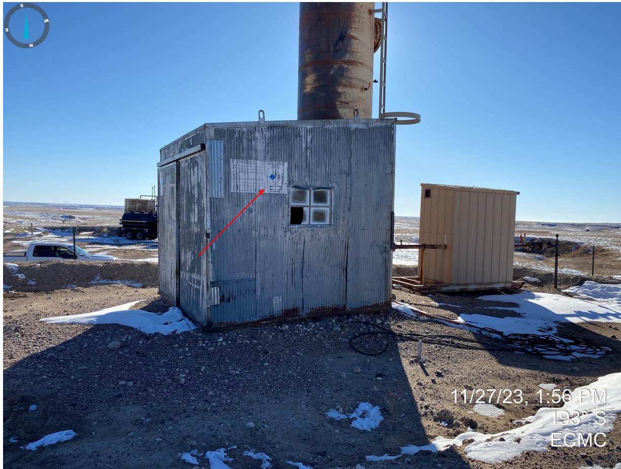
Photo 1. Sign and NFPA placard at vertical heater treater are not legible (e.g. peeling, faded, cracked).
