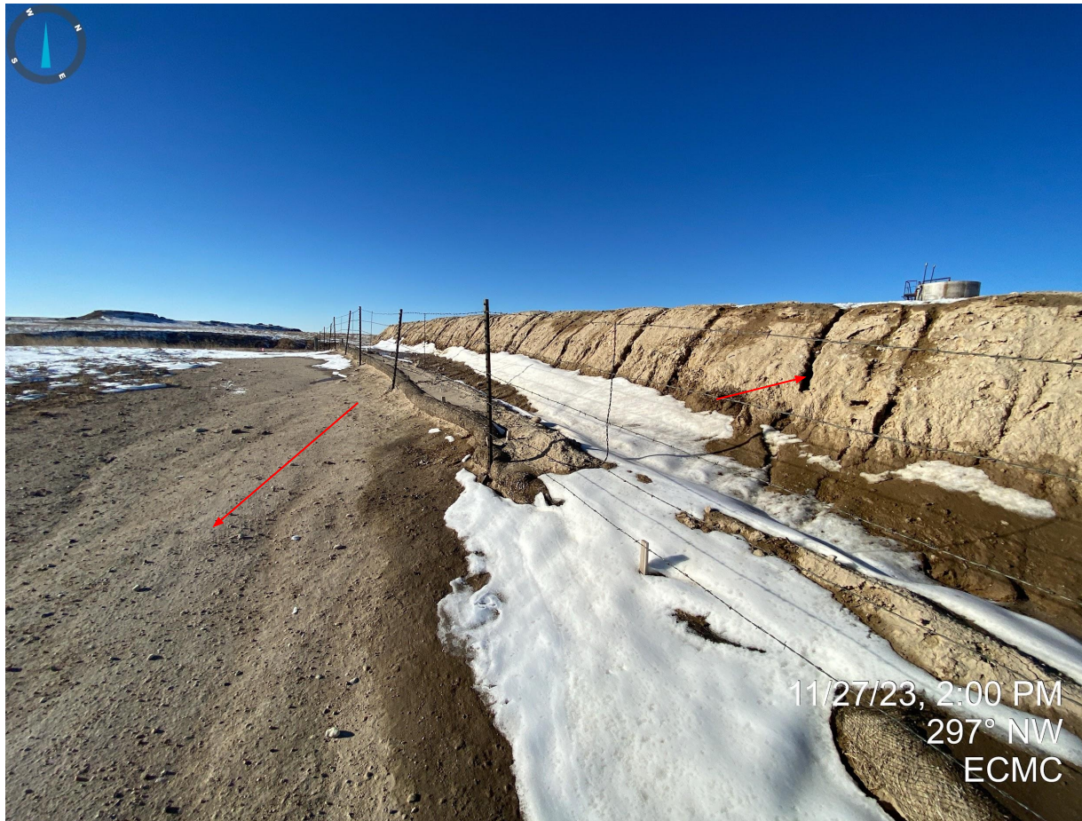
Photo 9. Taken near the southern portion of the location/pit. Exposed and bare soils south of the pit. No stormwater control measures or other stabilization BMPs of the exposed soils were observed during this inspection. Also pictured, erosion (e.g. rilling) occurring on the pit walls.
