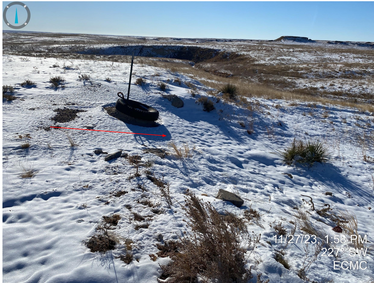
Photo 11. Areas northwest of the pit experiencing erosion degradation were previously documented and it does not appear any stormwater controls measures have been implemented and the unstabilized soils have not been repaired.
