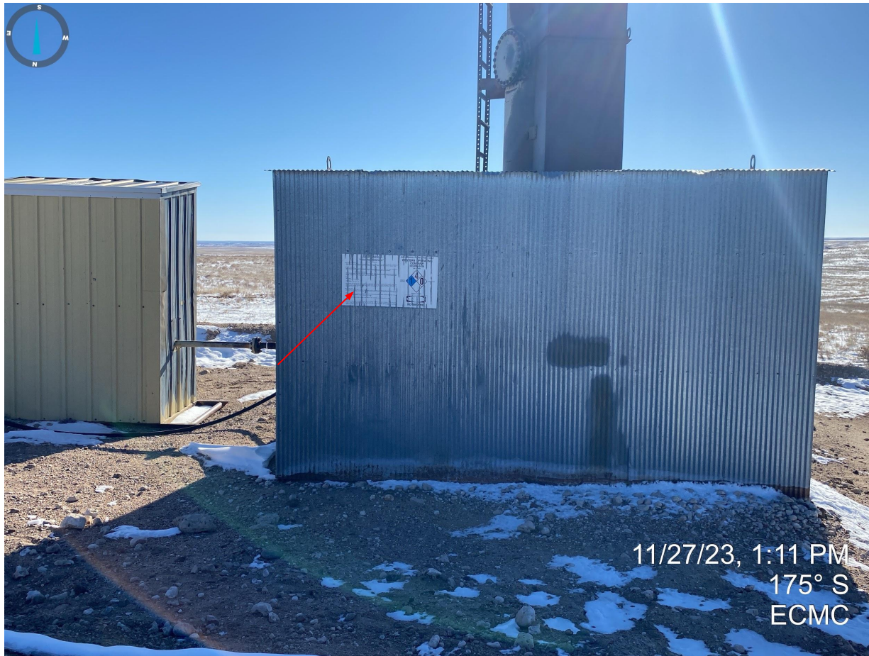
Photo 1. NFPA placard at separator shed is not legible (e.g. peeling, faded, cracked) and requires replacement.
