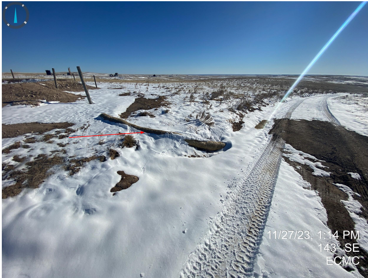
Photo 5. Taken from the western portion of the tank battery, photo illustrates stormwater control measure (straw wattle) that is not properly installed and is beginning to blow into the access road.
