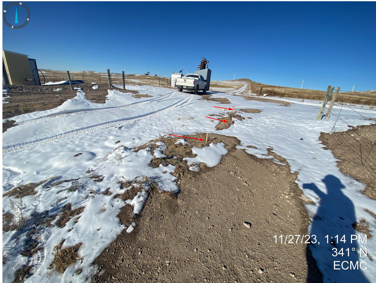
Photo 6. Continued from Photo 5. Photo illustrates stakes leftover from improperly installed straw wattle.
