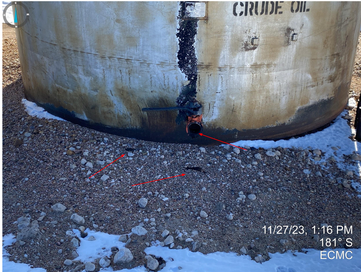
Photo 7. Stained soil observed near valve at AST within the tank battery.
