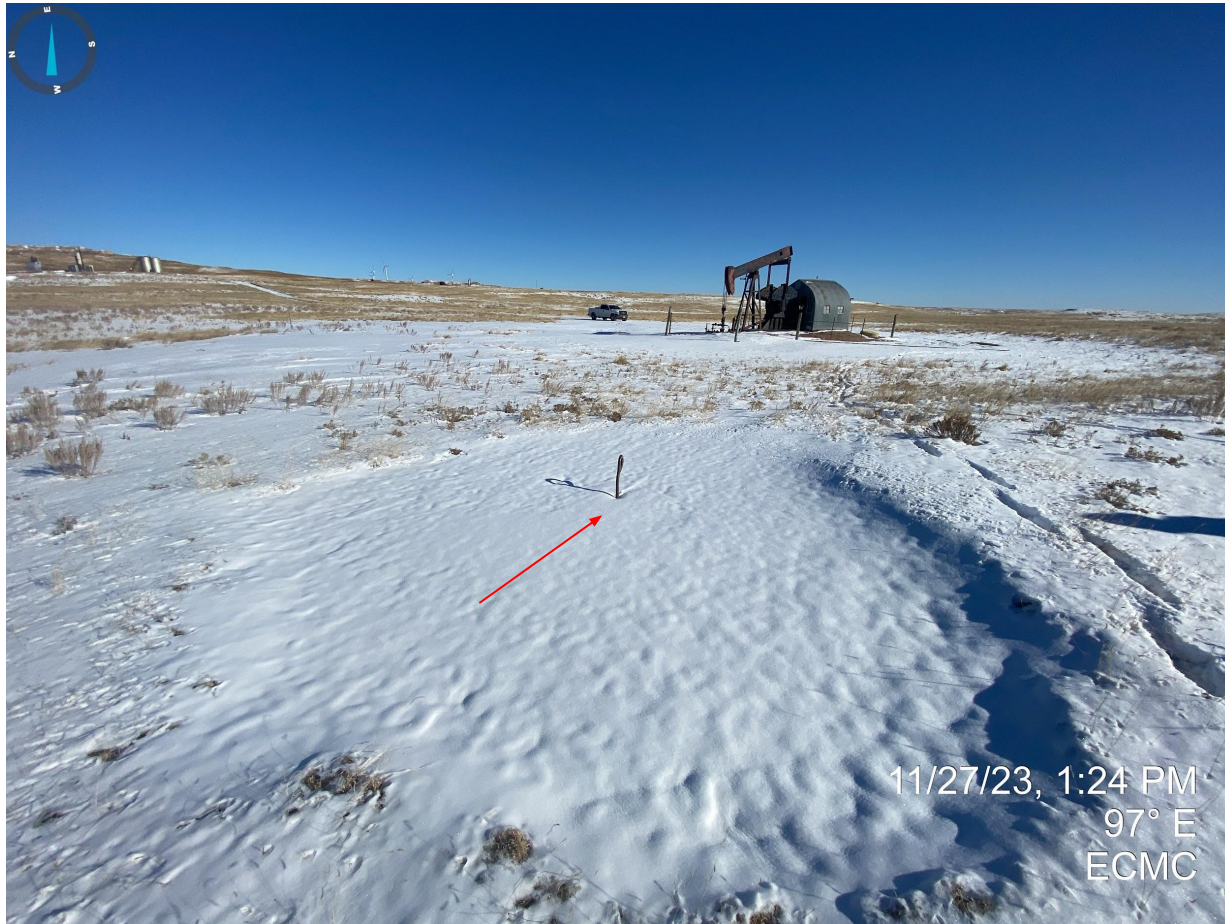
Photo 12. Northwest guyline anchor is not properly marked.
