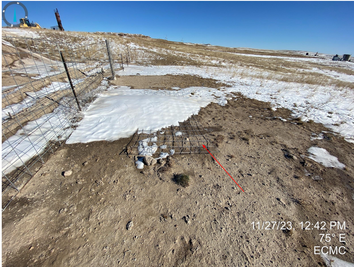
Photo 3. Cattle panel does not appear to be properly installed along with the other fencing; this is now considered unused equipment and either needs to be removed or reinstalled.
