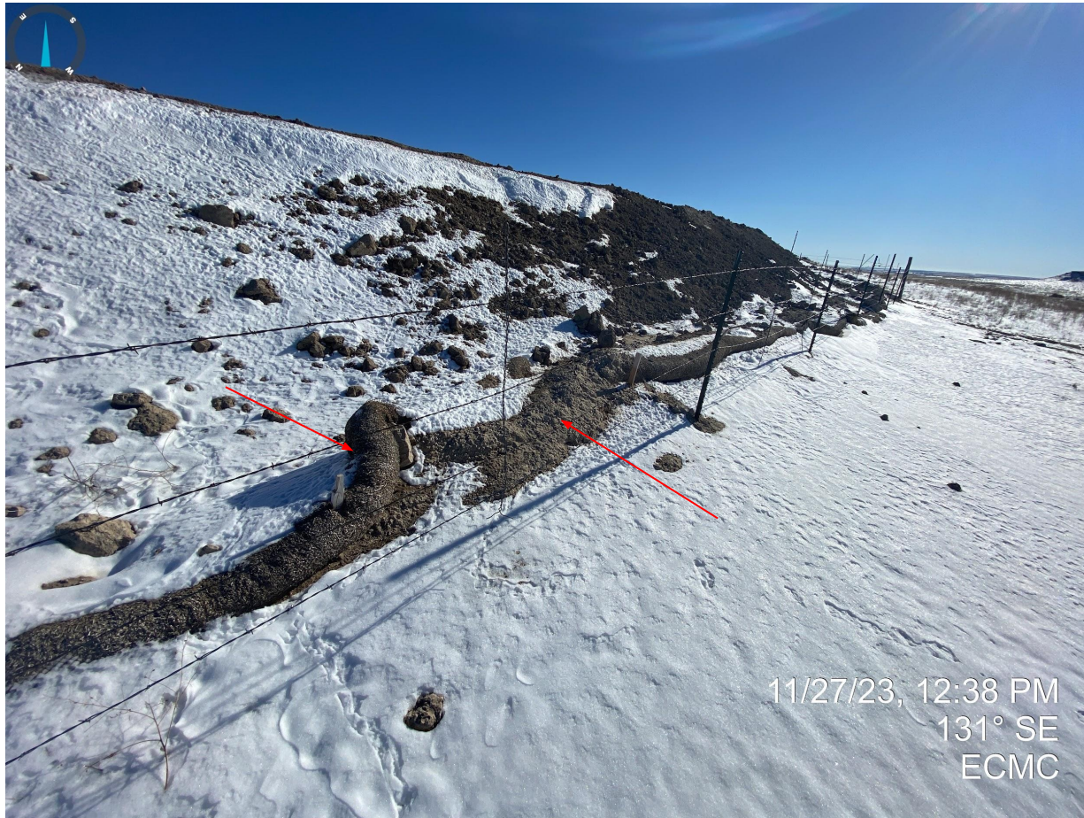
Photo 8. Taken from the western portion of the pit. Photo illustrates that straw wattles are inadequate as they are not installed properly and are degraded.
