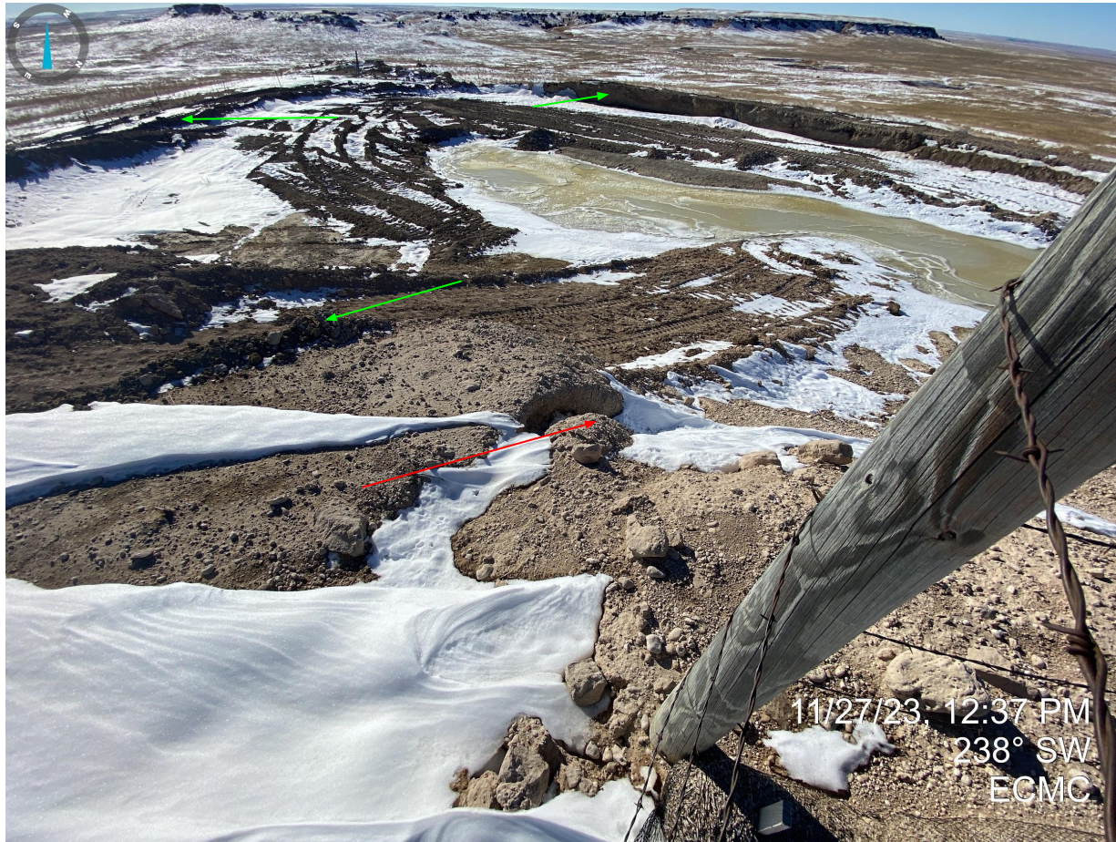
Photo 4. Taken from the eastern side of the pit. Photo illustrates erosion degradation (e.g. gullying with red arrow) that does not appear to have been repaired or stabilized, and no apparent stormwater control measures to prevent further erosion. Additionally, recent earthwork associated with soil sampling has left much of the pit with unstabilized/unconsolidated materials that can become a source of pollution itself (represented by green arrows).
