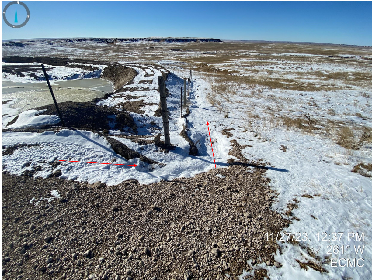
Photo 7. Taken from the northeastern portion of the pit. No apparent stormwater management work appears to have been performed since the previous inspection(s) to stabilize the eroded portions observed here.
