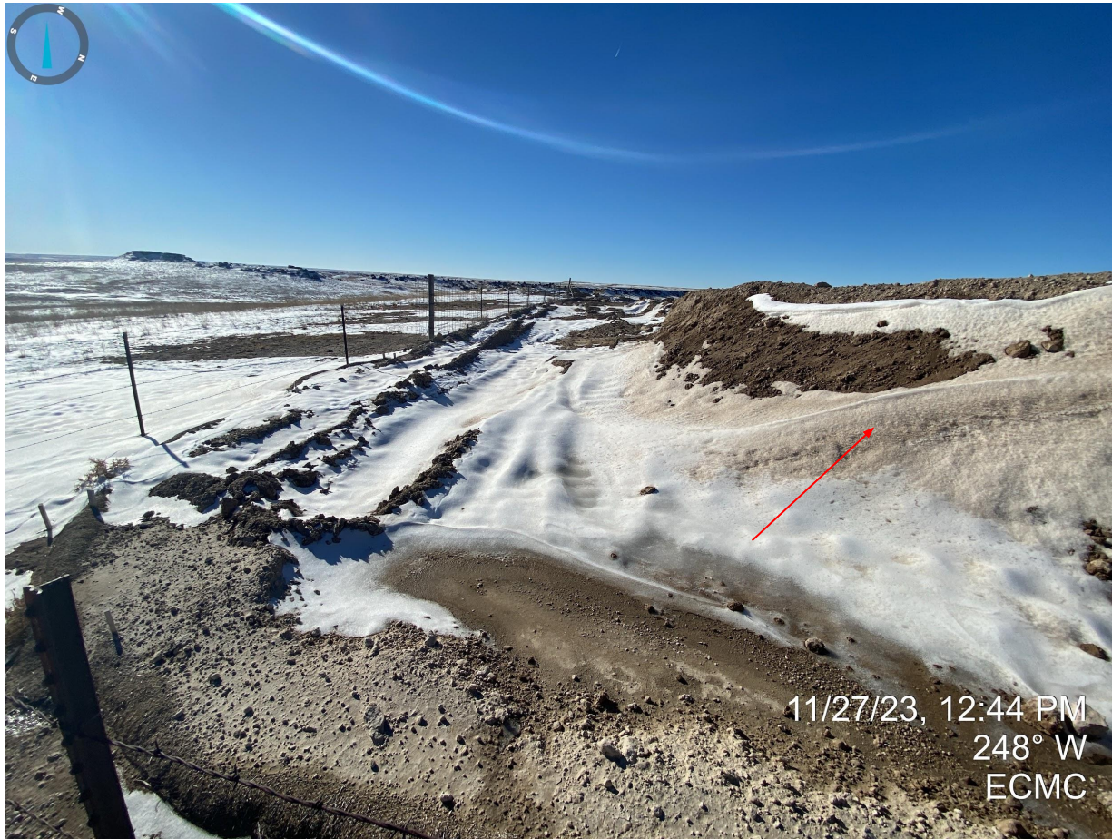
Photo 15. Continued from Photo 14. Red arrow illustrates dust on snow, indicative of wind erosion, from unconsolidated materials.
