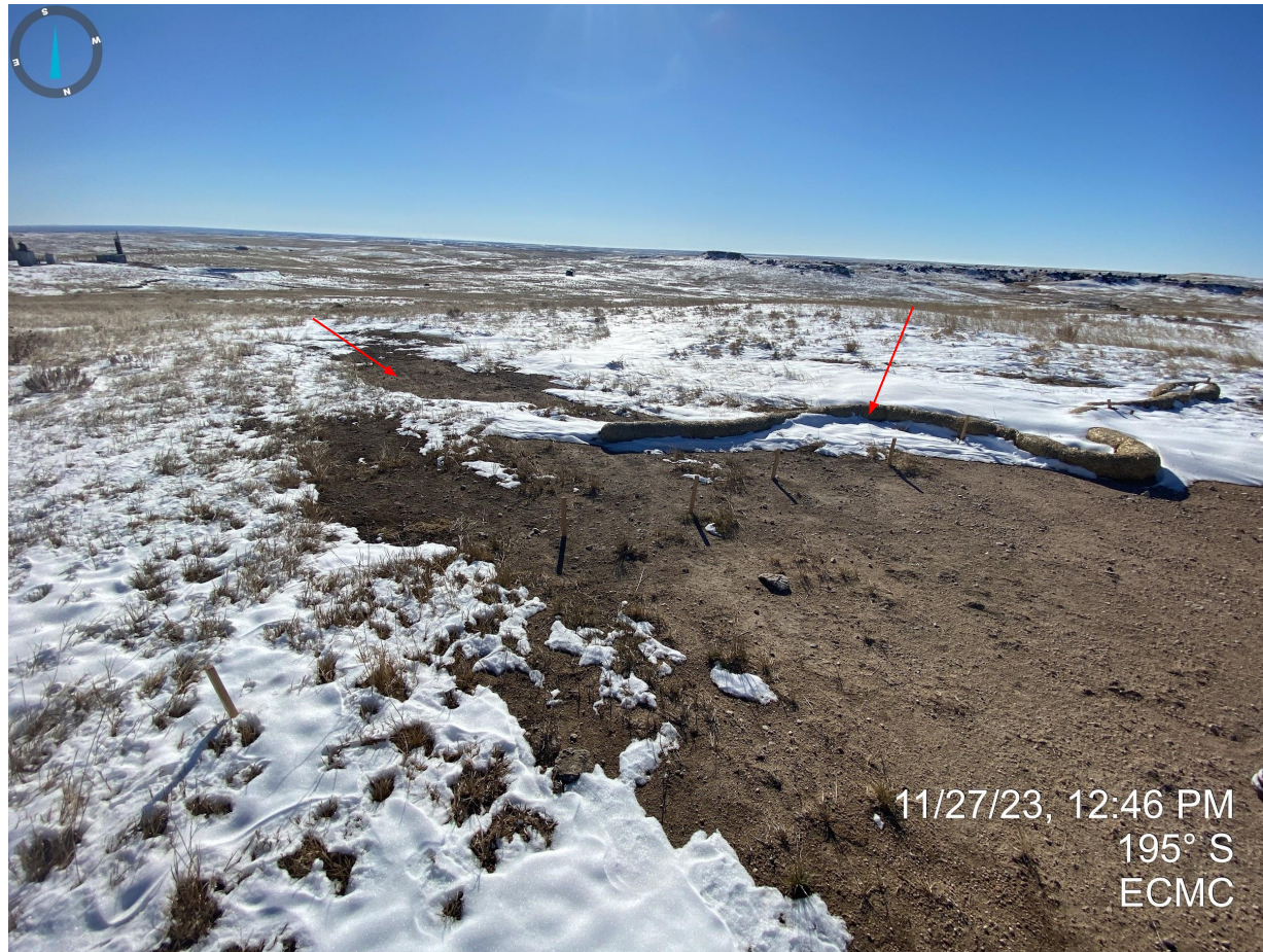
Photo 19. Taken near the vertical heater treater. Photo illustrates that straw wattles are not properly installed and bare/exposed soils are not properly stabilized.
