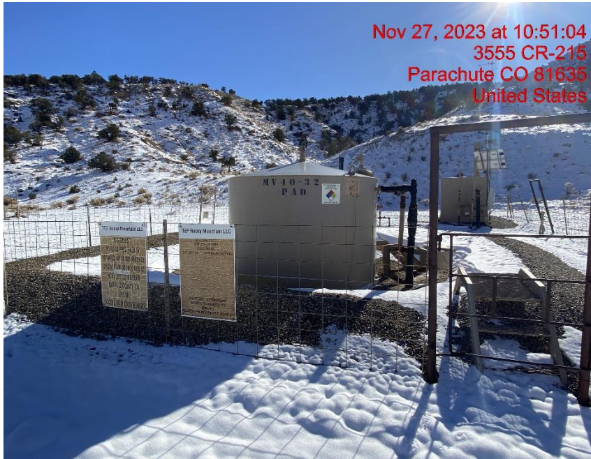
Tank Battery – Photo #07696
