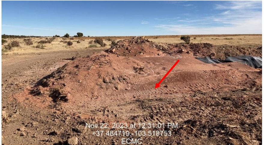
**Photo 7 – Drill Cuttings with no Liner or containment**
