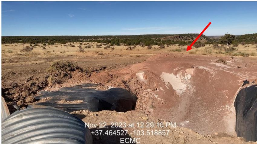
**Photo 11 – Drill Cuttings Trench and Drill Cuttings**
