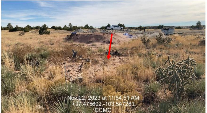
**Photo 7 – Drill Cuttings not properly stored**
