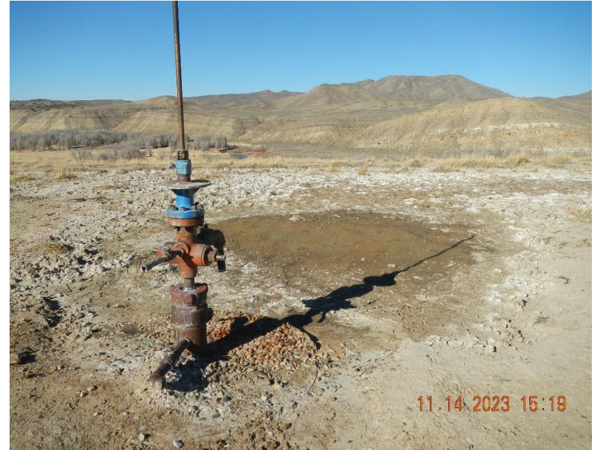
BM Federal #13-12 well head and impacted area.
