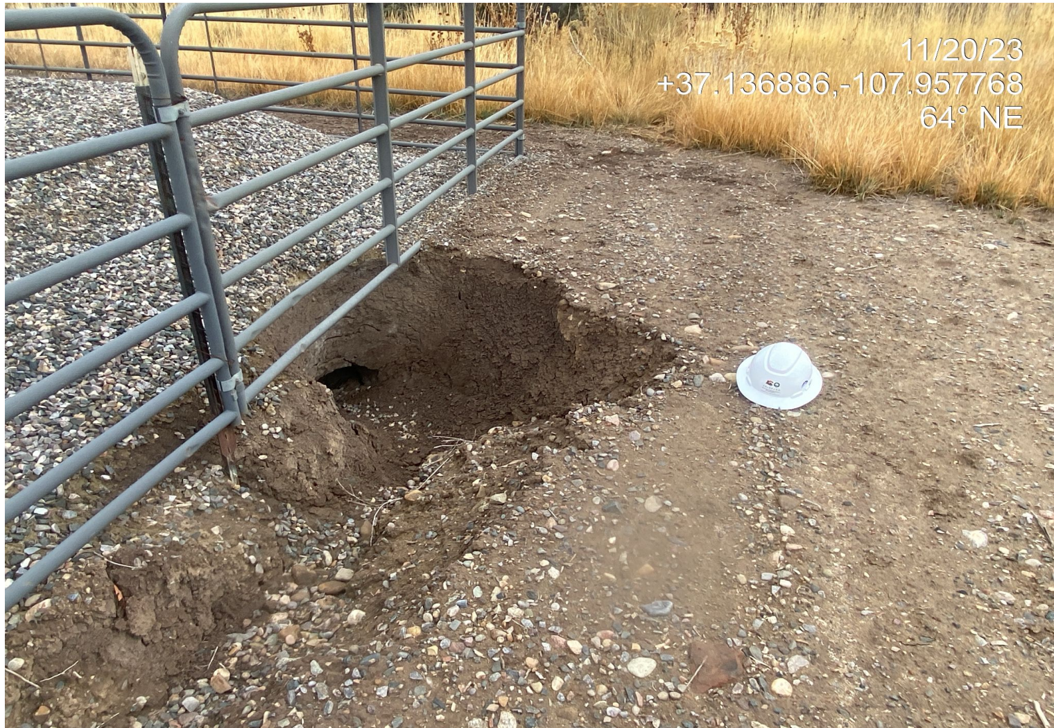
Photo 2. Large erosion feature observed on the disturbance. Approximately 3 feet deep.
