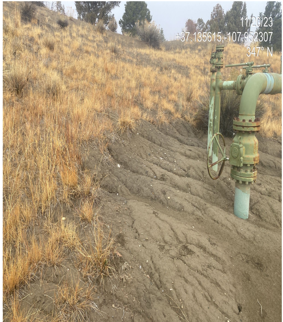
Photo 3. Rill erosion observed in the northern interim reclamation area at the base of the cut slope.
