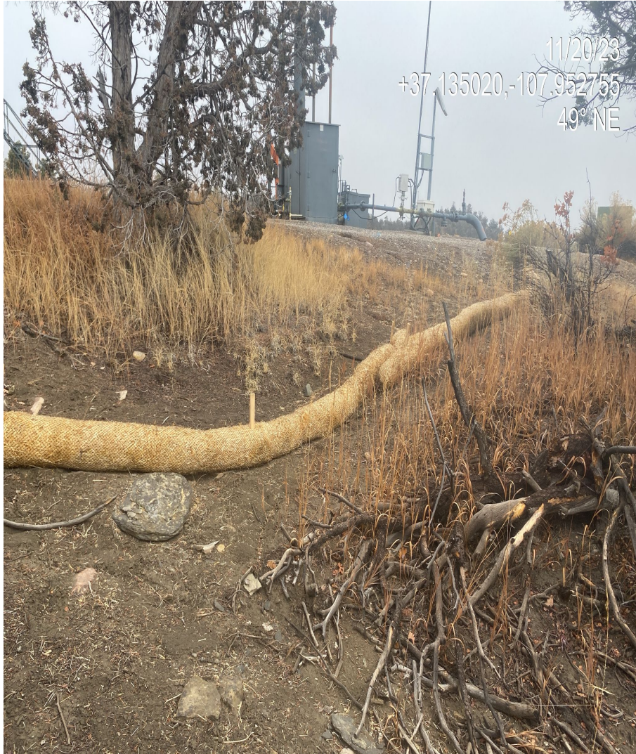
Photo 4. View of wattles that are not installed properly installed in the western interim reclamation area.
