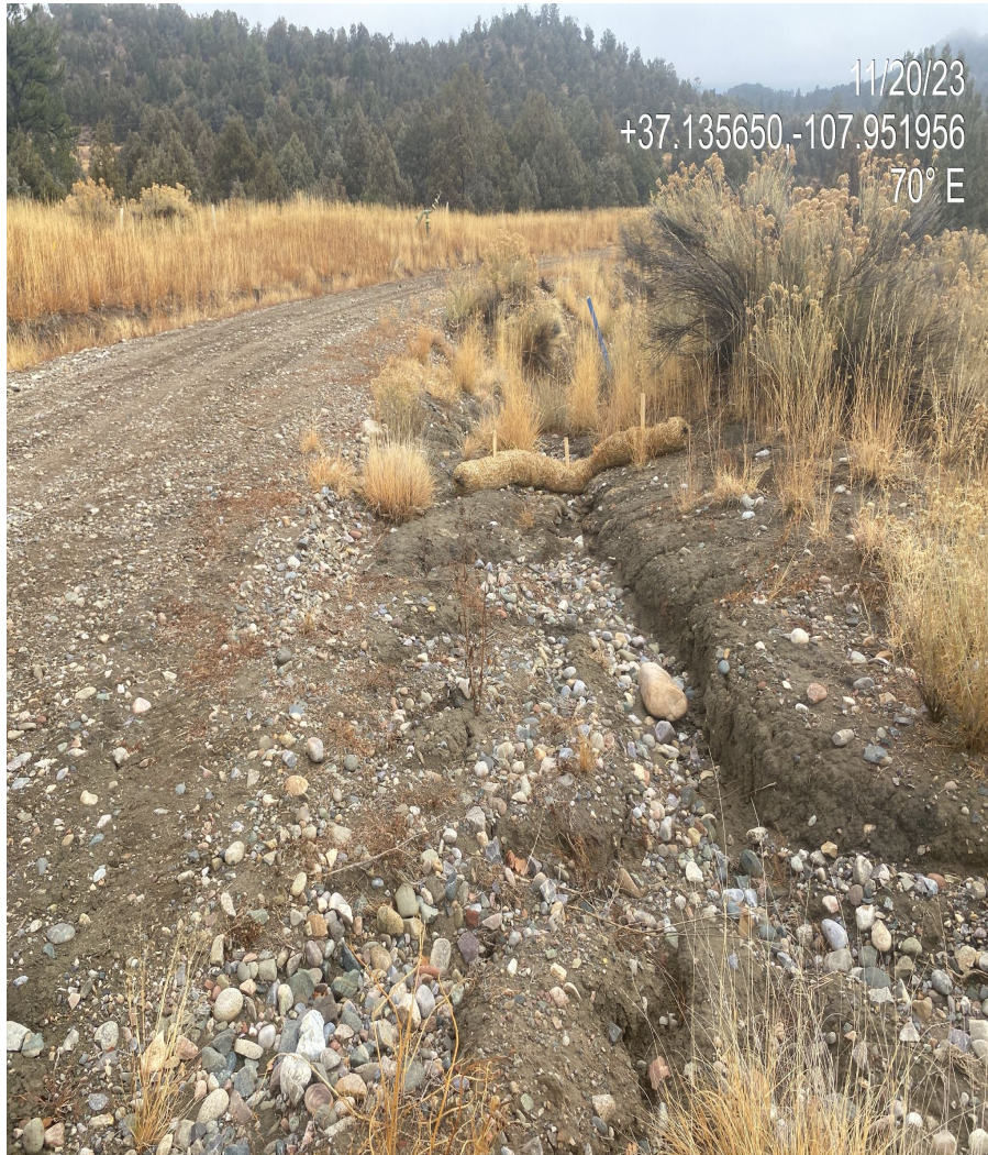
Photo 2. View of the erosional channel that remains along the access road. Stormwater BMPs installed are not functioning.
