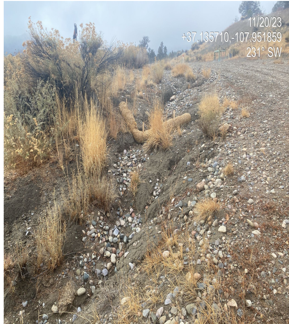
Photo 2. View of the erosional channel that remains along the access road. Stormwater BMPs installed are not functioning.
