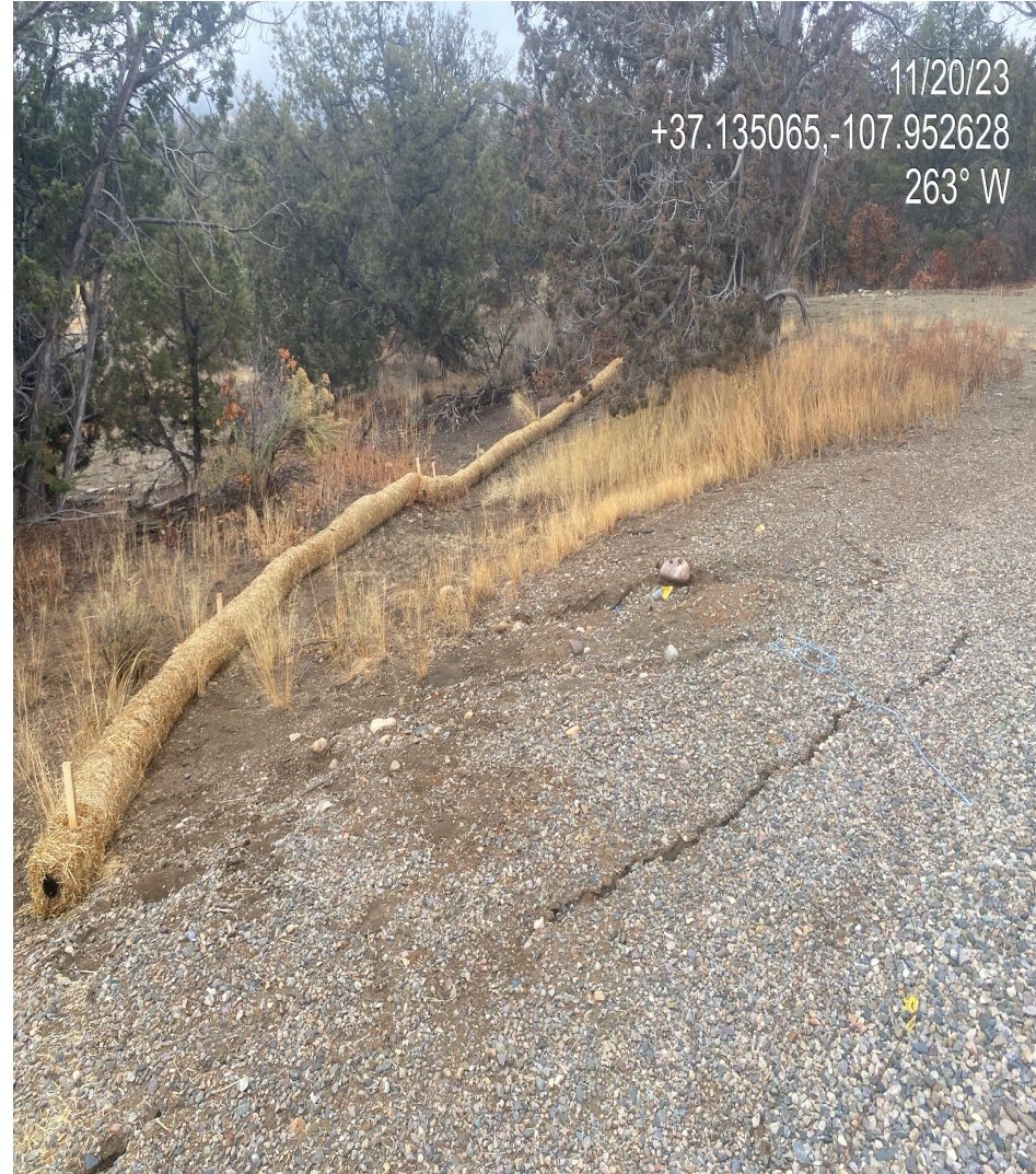
Photo 4. View of wattles that are not installed properly installed in the western interim reclamation area.
