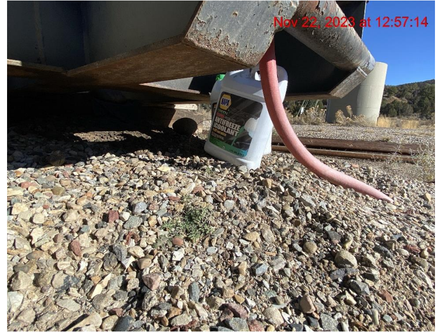
Antifreeze Stored on Location (No NFPA label or secondary containment) – Photo #07623
