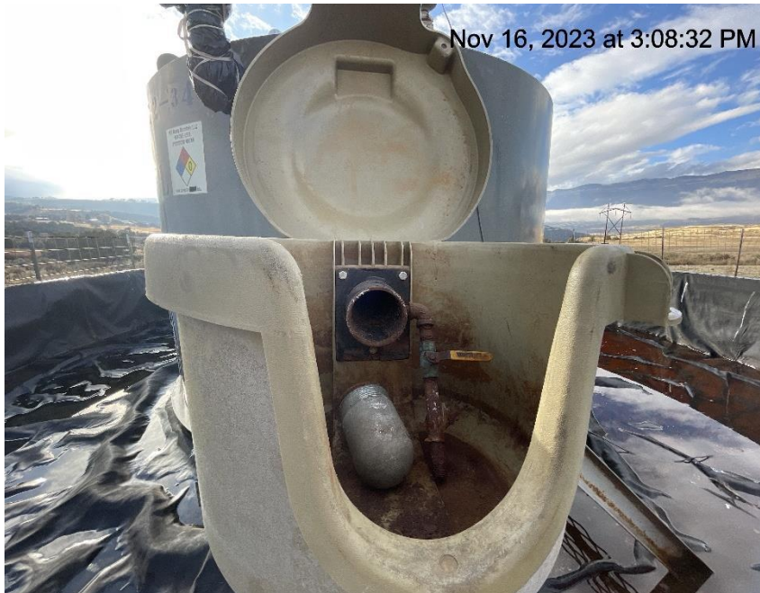
Photo # 7007 From inspection 708902256 conducted on 11/16/2023 Open ended load line
