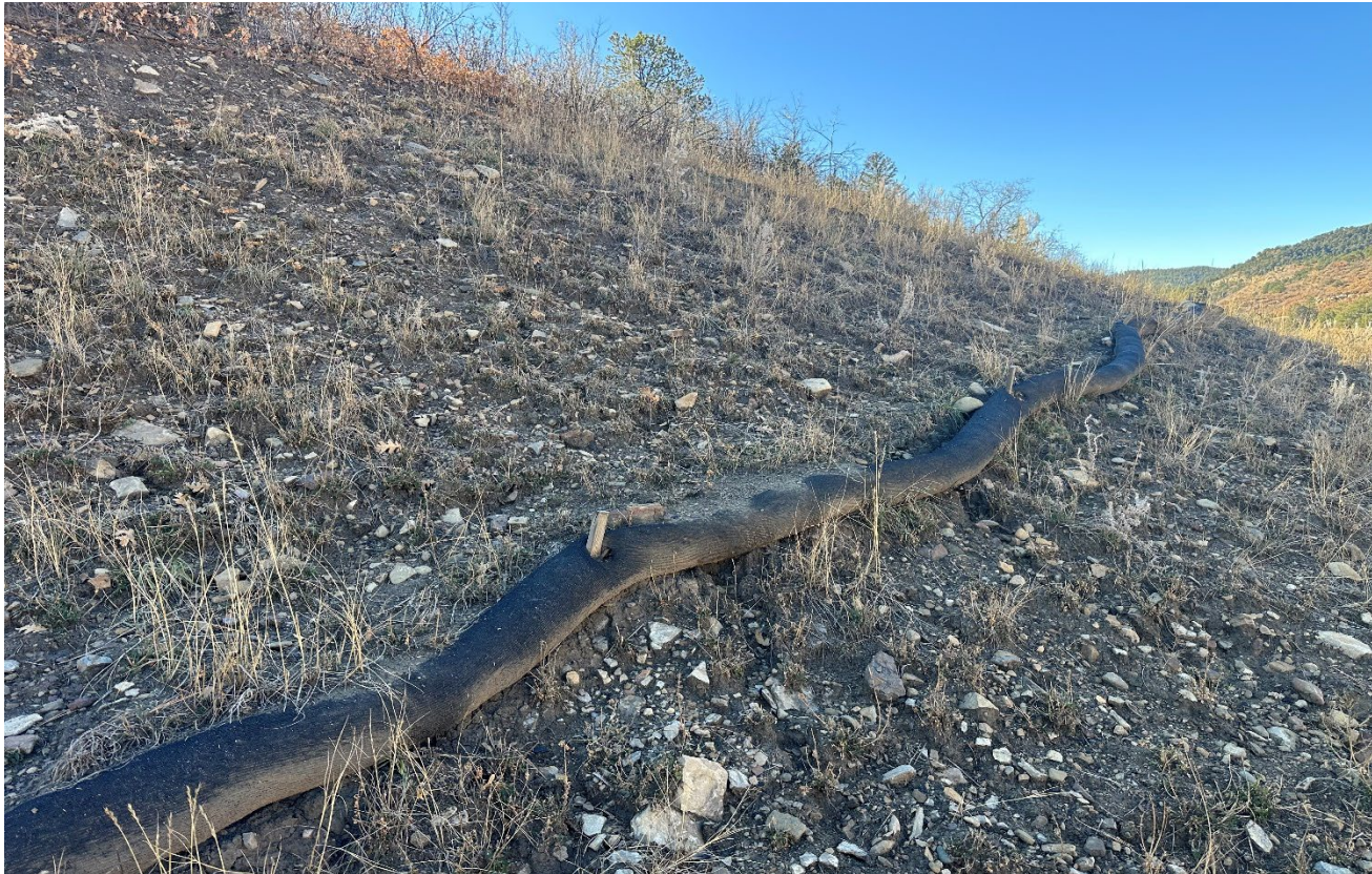
Photo 6. Facing toward the upper center of the location. This area approximately 15'x15' has less vegetation cover. The erosion wattles will need to be removed for final reclamation.
