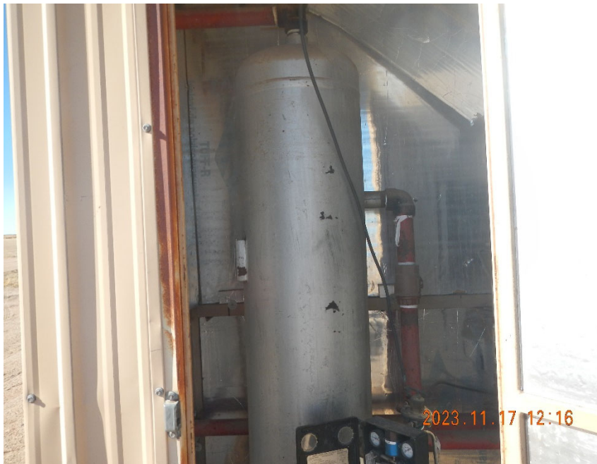
5. Vertical separator inside shed.
