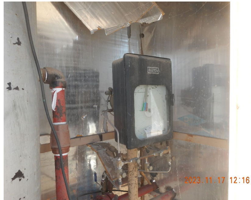
6. Gas meter run inside shed.
