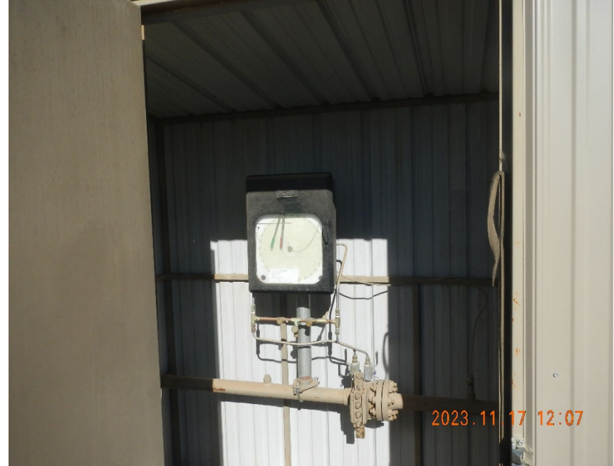
6. Gas meter run inside meter shed at remoted location.
