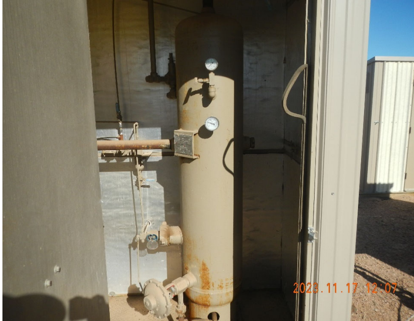
5. Vertical separator inside separator shed at remote location.
