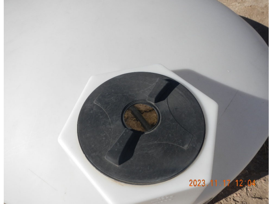
10. Produced water tank hatch with missing cap.
