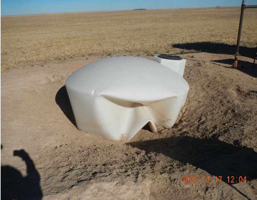
9. View of produced water tank with dented side.
