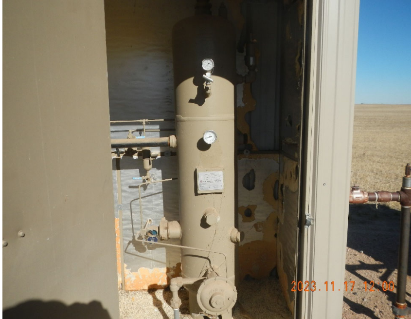
5. Vertical separator in separator shed.
