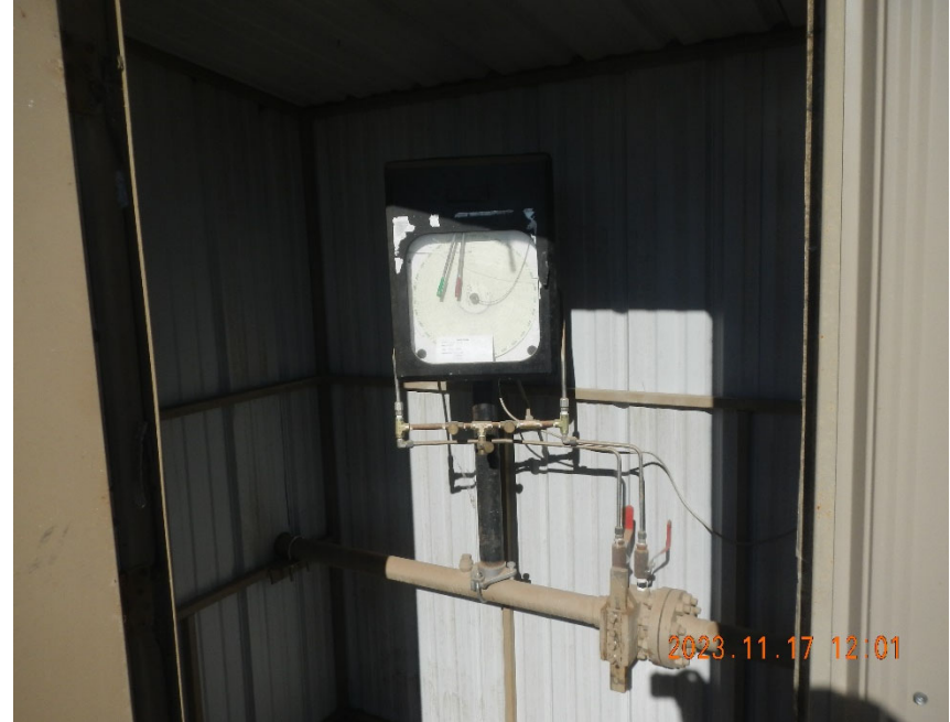
6. Gas meter in meter shed.
