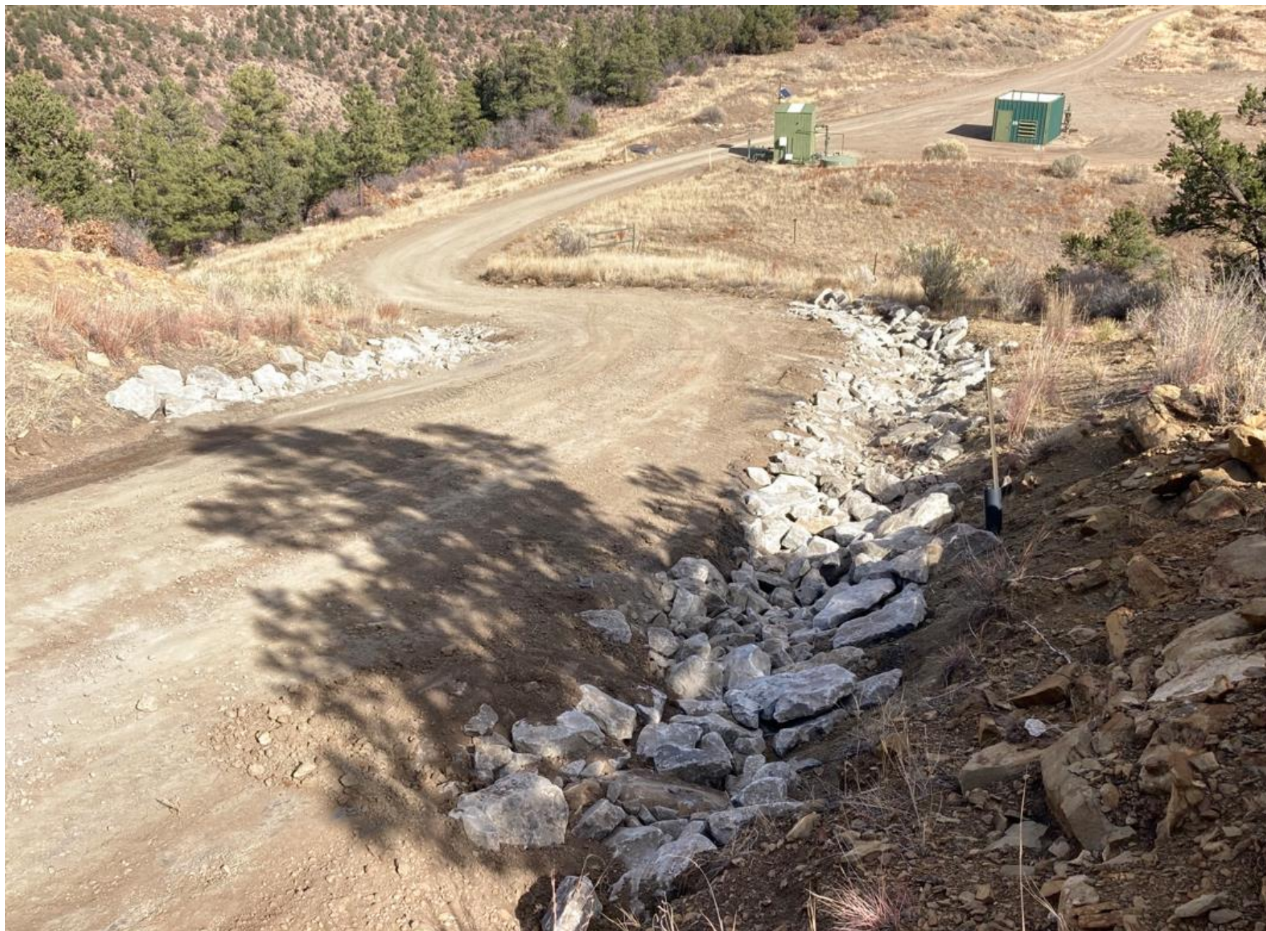
PHOTO 2: THE ROCKED DIVERSION DITCHES ALONG SIDE THE MAIN ACCESS ROAD LEADING TO LOCATION.
