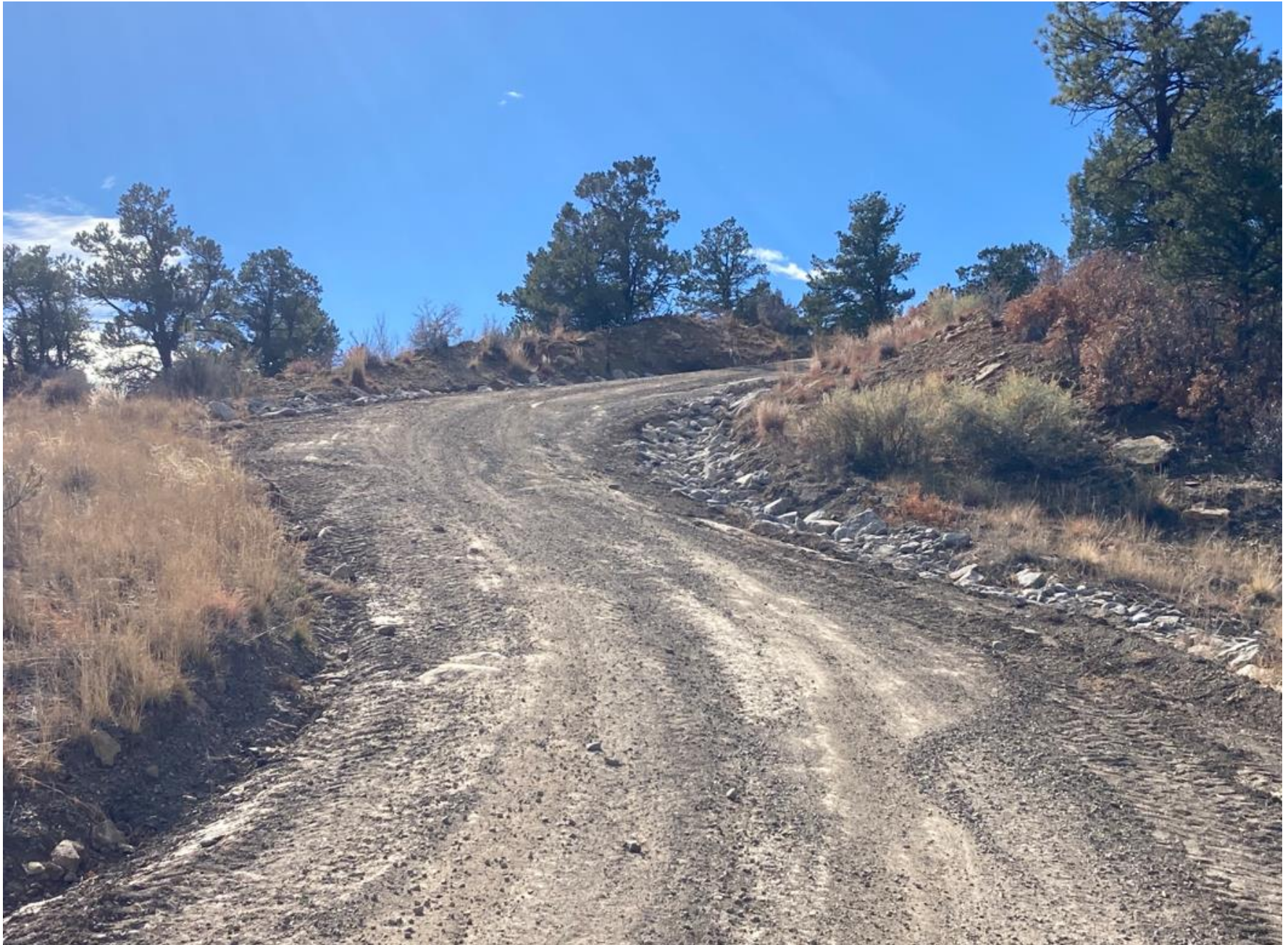
PHOTO 1: THE MAIN ACCESS ROAD LEADING TO LOCATION HAS BEEN BLADED AND CROWNED TO DIRECT STORMWATER TO THE ROCKED DIVERSION DITCHES. TURN OUTS WERE ALSO ESTABLISHED.
