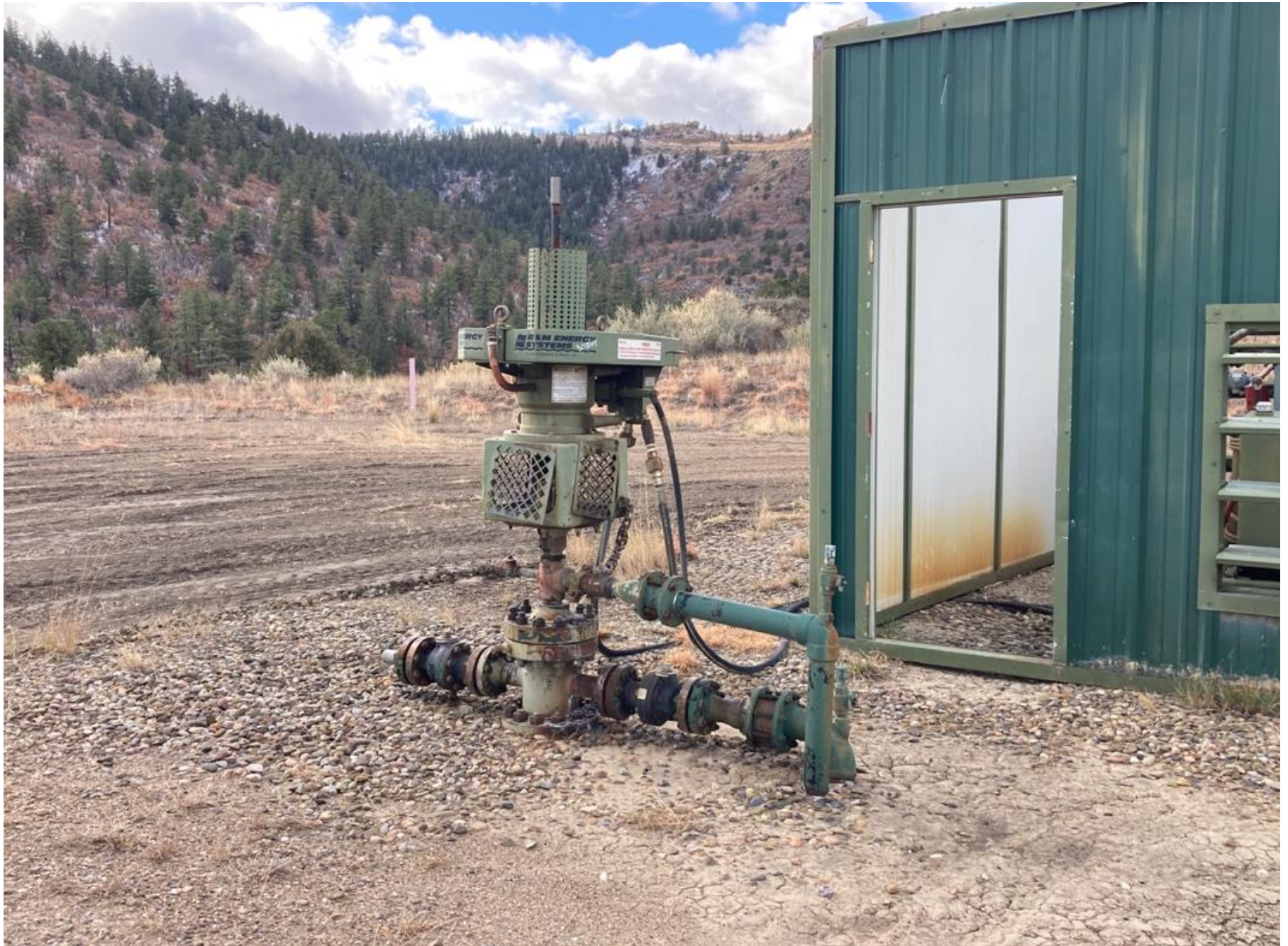
PHOTO 3: THE WATER LEAK AT THE WELL HEAD WAS STOPPED IMMEDIATELY AND MECHANICAL MAINTENANCE WAS PERFORMED. THE STAINED SOIL WAS REMOVED FROM LOCATION AND FRESH GRAVEL ADDED TO THE WELL PAD. THE SELF INSPECTION PROCESS HAS BEEN REVIEWED.
