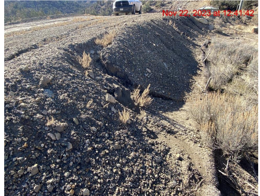
Erosion Transporting Sediment Off Location – Photo #07612
