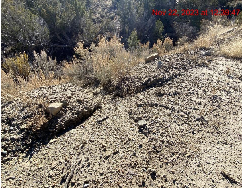
Erosion Transporting Sediment to Watershed – Photo #07606
