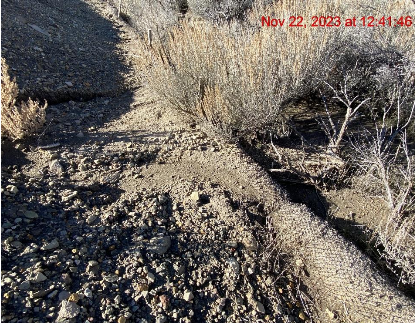
Insufficient Waddle BMP – Photo #07613
