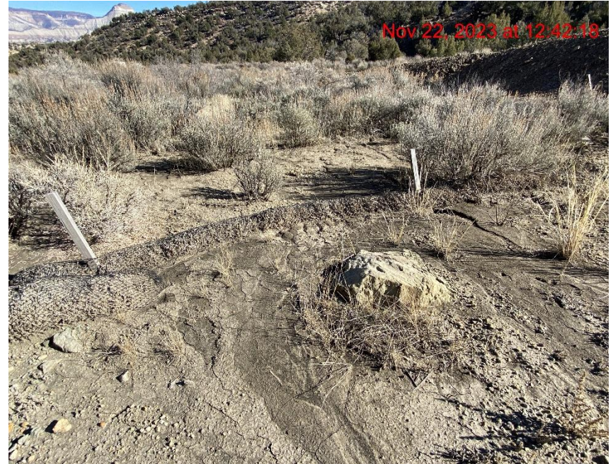
Insufficient Waddle BMP – Photo #07615
