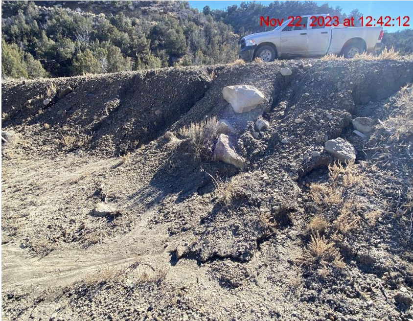
Erosion Transporting Sediment Off Location – Photo #07614
