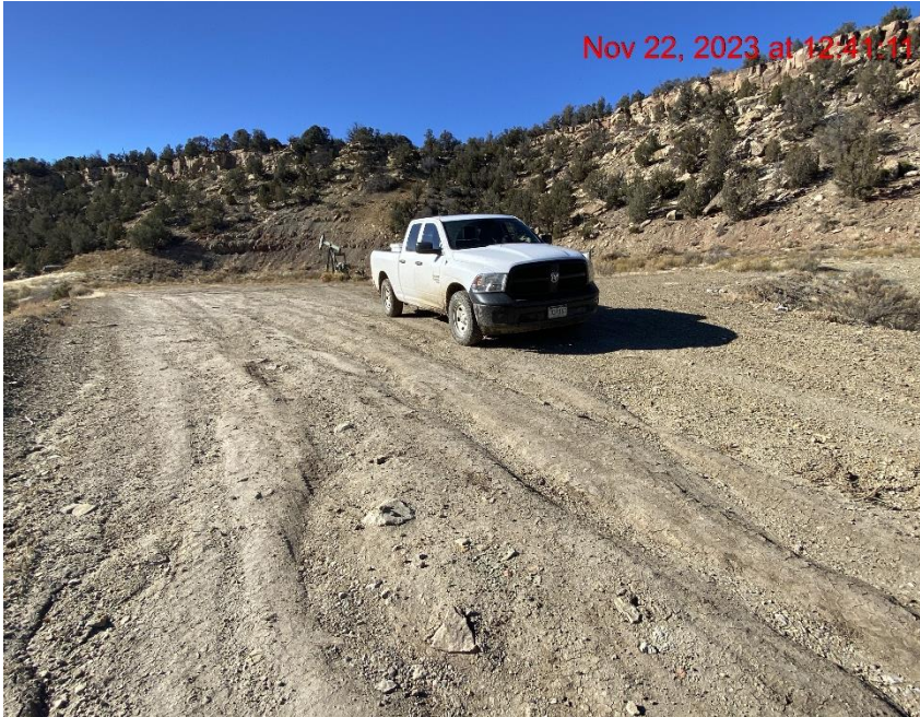
Insufficient Vehicle Tracking BMPs at Location Entrance/Exit – Photo #07610
