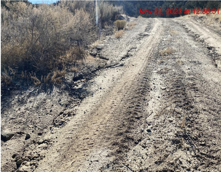
Insufficient Erosion Control/Rill Erosion on Access Road – Photo #07600
