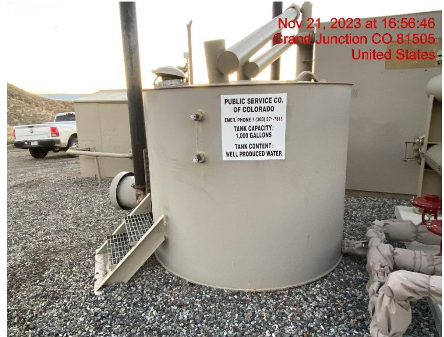
No Secondary Containment – Photo #07581
