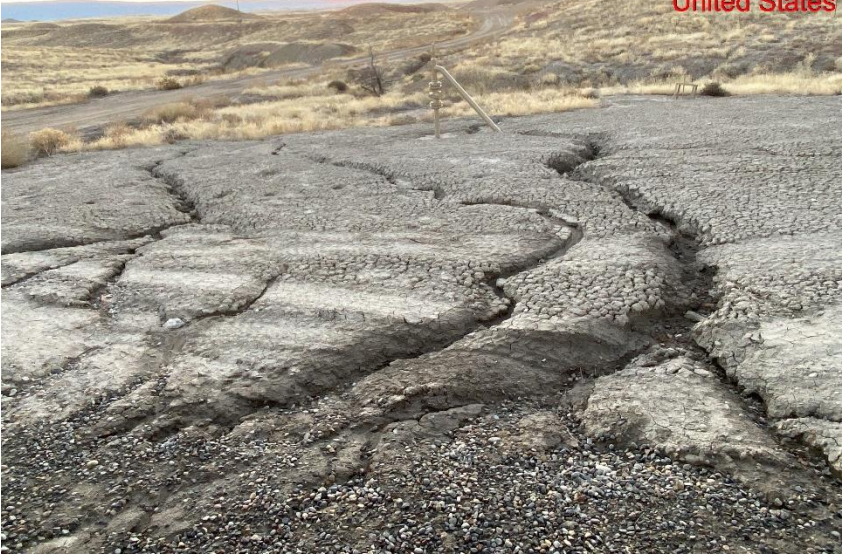
Rill Erosion Transporting Sediment Off Location – Photo #07579
