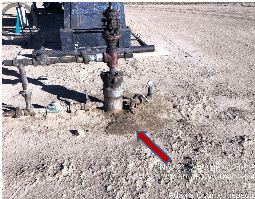
Photo #6 stained soil around well head.
