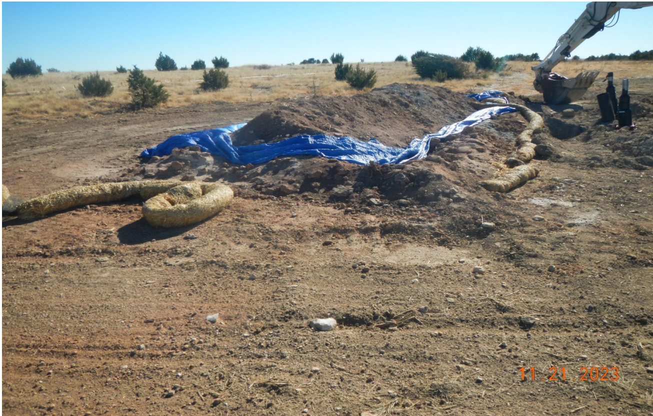
Photo 3. Facing southeast toward the drill cuttings pile. The pile is not properly stored with containment. It appears the drill cuttings were used as berms and wattles are not maintained around the pile.
