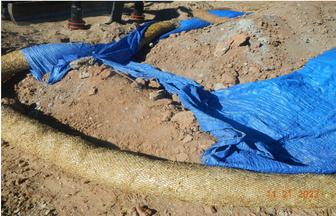
Photo 6. The material used for a berm is the same color as the drill cuttings. The cuttings pile is not properly stored with sufficient containment..
