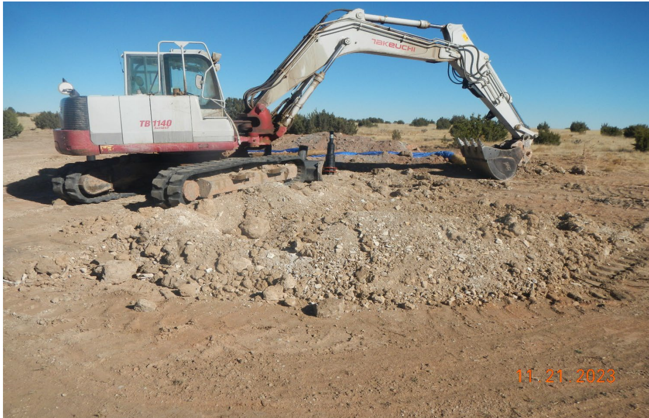
Photo 7. It appears the area of the wellhead was excavated and subsoils were brought to the surface. The subsoils have the light colored rock material shown in the pile next to the excavator.
