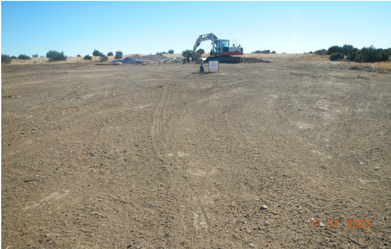
Photo 2. Facing southeast toward the Red Rocks #35-08 drill site. It appears soils have been graded however, soils are compacted from heavy equipment and will need to be properly decompacted.
