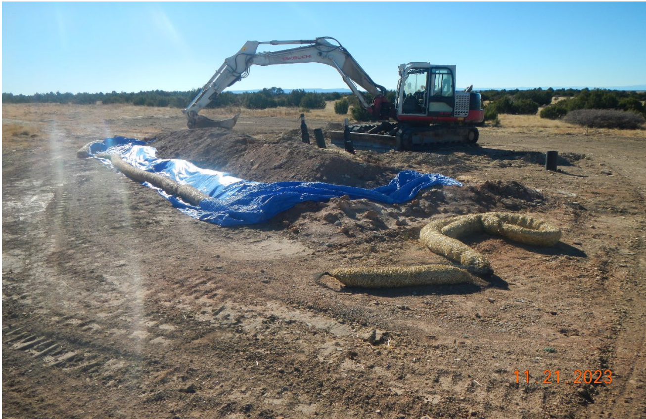
Photo 5. Facing southeast toward the drill cuttings pile. The pile is not properly stored with containment. It appears the drill cuttings were used as berms and wattles are not maintained around the pile.
