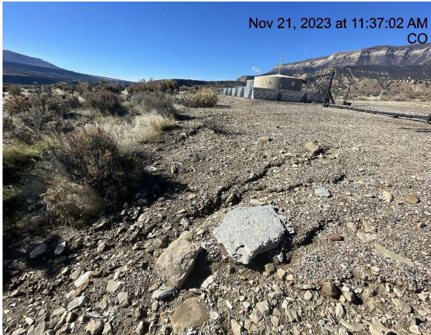
Photo # 7231 Erosion & transport of sediment off location
