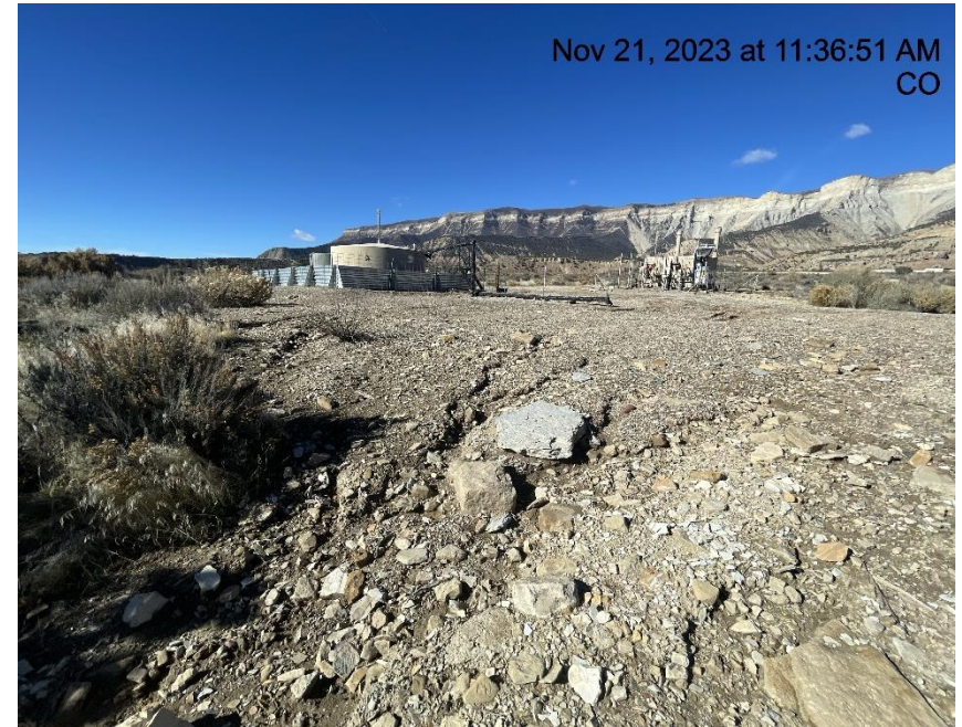
Photo # 7230 Erosion & transport of sediment off location
