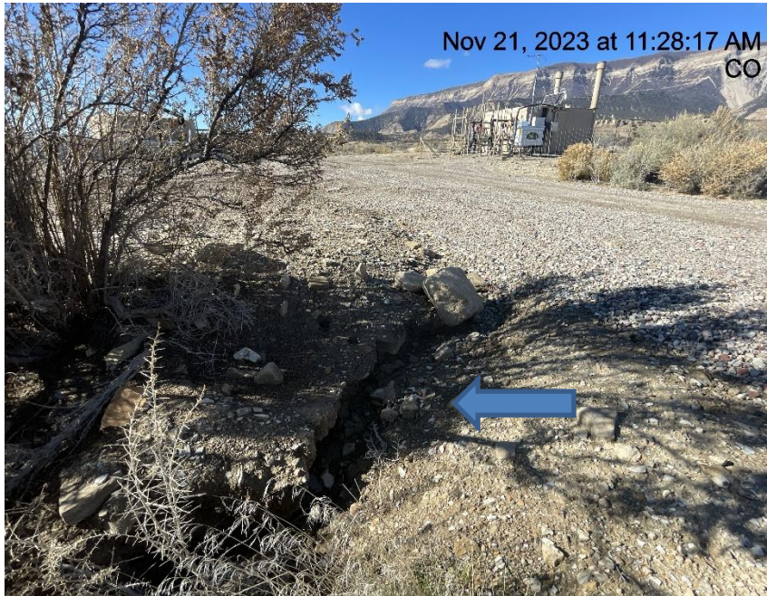
Photo # 7227 Erosion & transport of sediment off location
