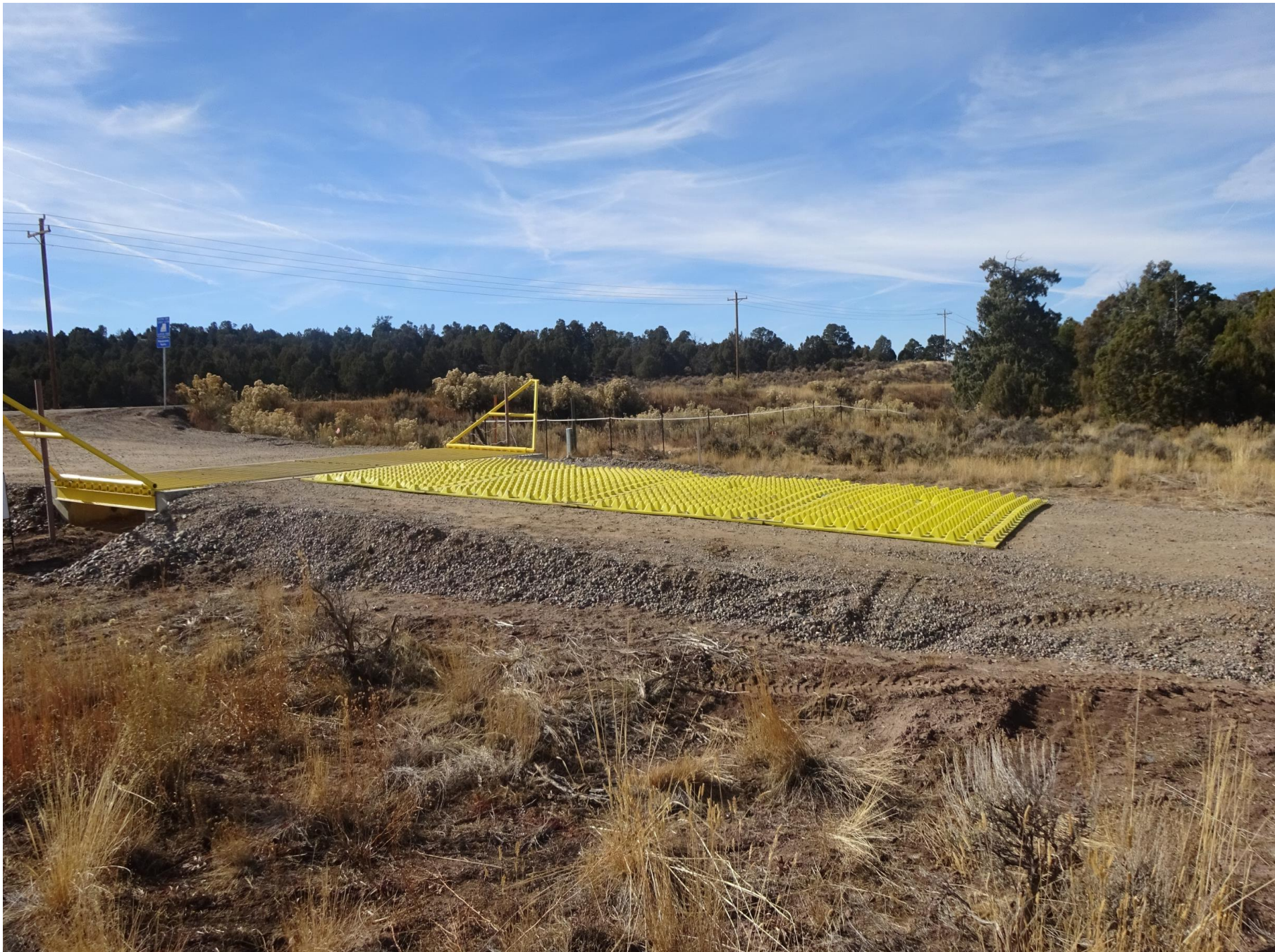
NueVida Resources, LLC Ardourel 33081718 Facility ID: 484496 South entrance from CR-318 onto lease road. Cattleguard and Tracking Mats. (looking southwest)
