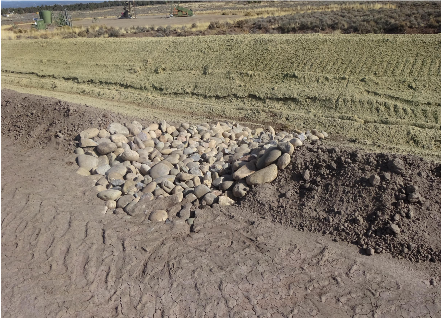
NueVida Resources, LLC Ardourel 33081718 Facility ID: 484496 East side of Water Pad Drainage/cobble (rip-rap) area along Water Pad road (looking northeast)
