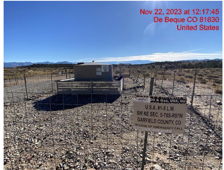
Tank Battery – Photo #07587
