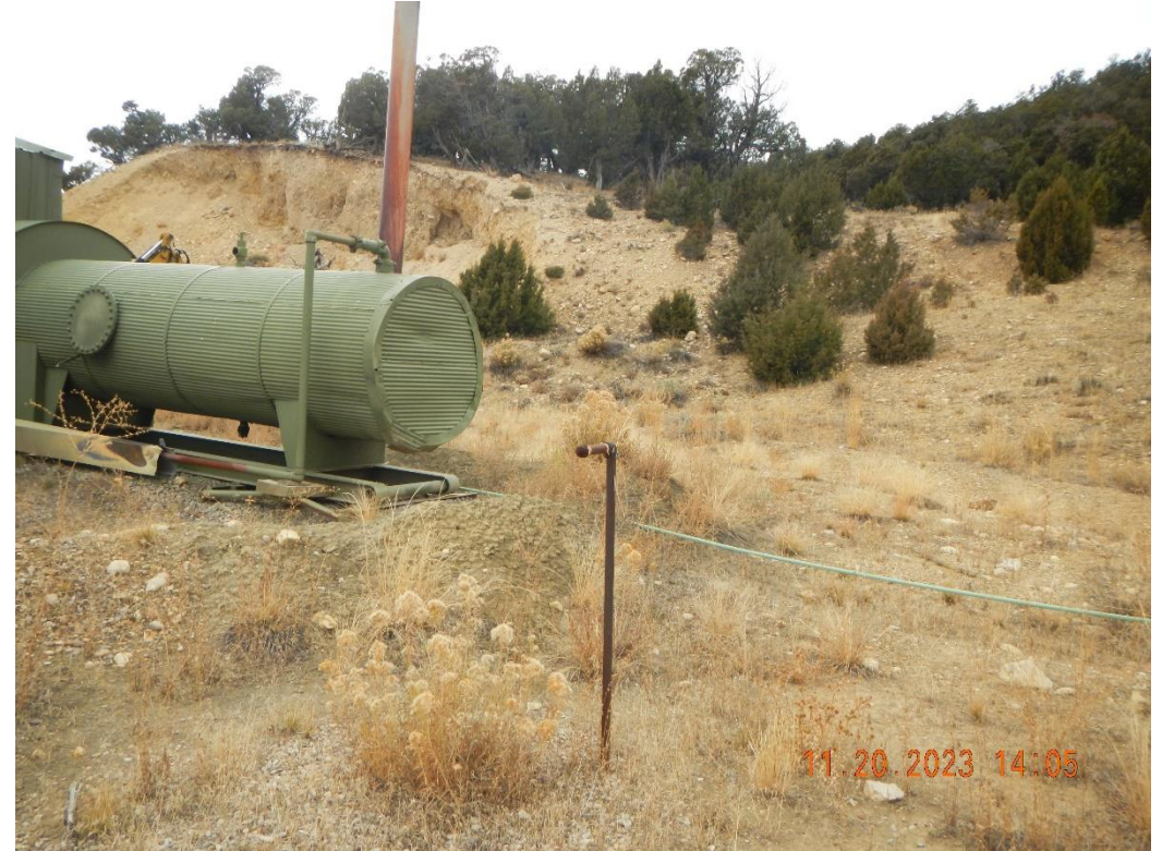
Unused 1" riser at separation equipment.
