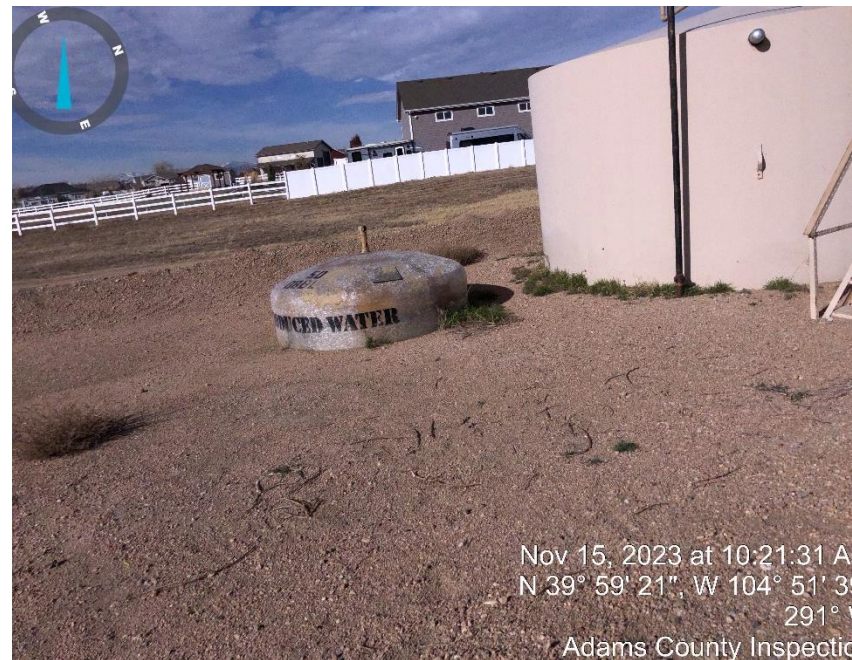
Photo #2 P/W tank.
