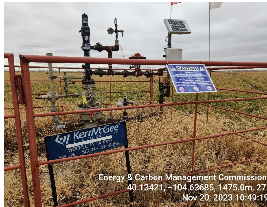
Photo 6: SI Wellhead, WEEDS
