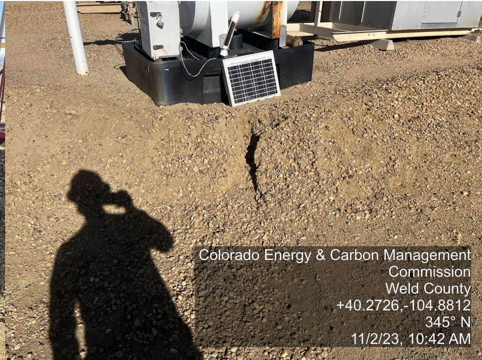
Photo 2. The photo was taken on the South side of the tank battery location facing North. The photo illustrates erosion creating rills in the road mix pad.
