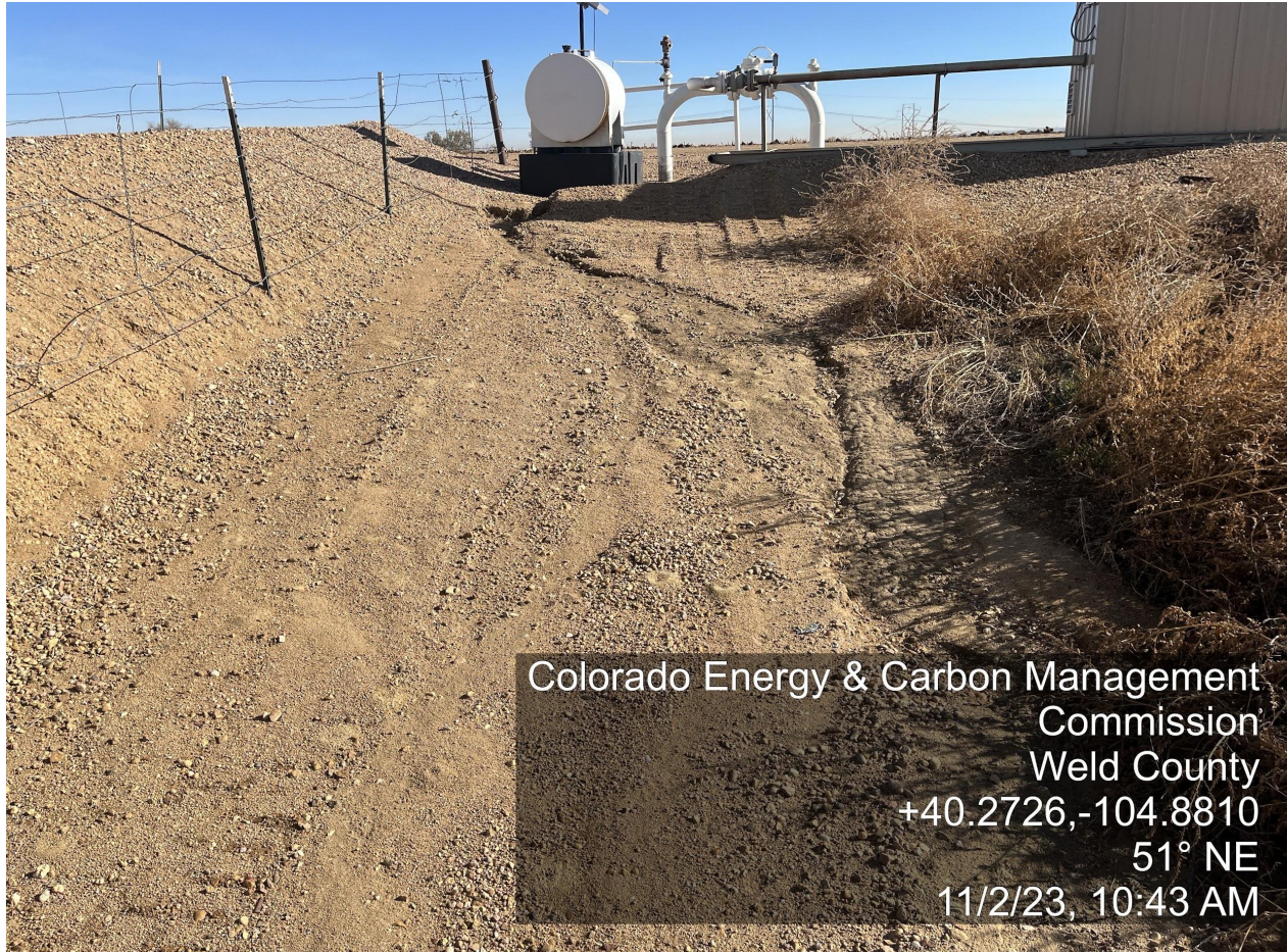
Photo 5. The photo was taken at the South side of the tank battery location facing Northeast. The photo illustrates large amounts of rilling and undesirable vegetation.
