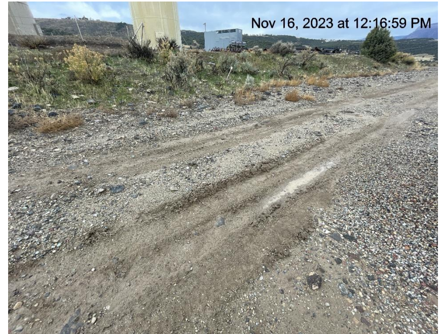
Photo # 6902 Lack of stabilization/compaction
