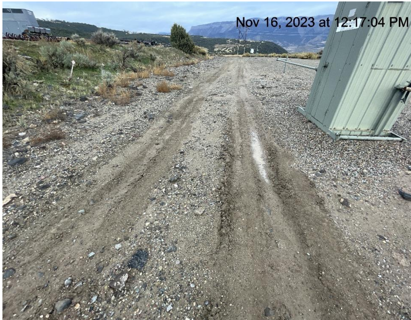
Photo # 6903 Lack of stabilization/compaction
