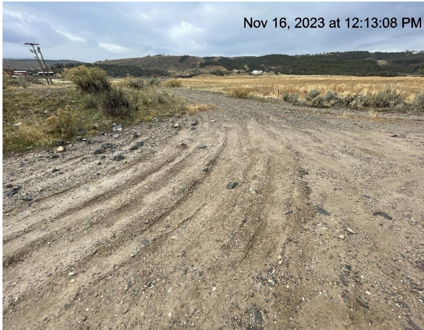
Photo # 6901 Lack of stabilization/compaction
