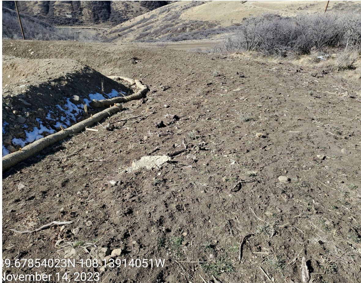
Photo 14: Photos taken from the north end of the Location. Photo shows erosion logs are no longer in proper functioning condition. Photo also shows BMPs to minimize erosion, degradation and sediment transport at the topsoil stockpiles are no longer in proper functioning condition; hydromulch has degraded
