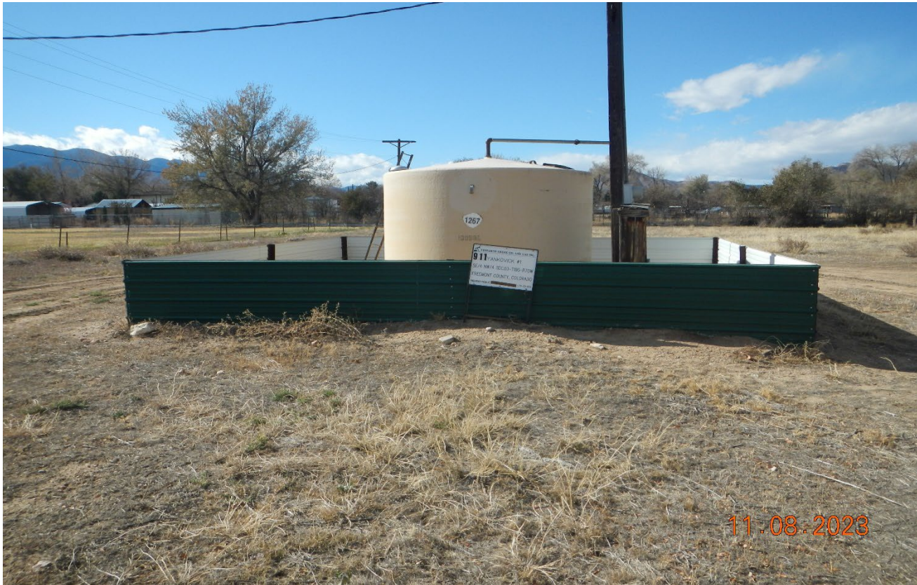
Photo 1. Facing west toward the tank battery. It looks like the capacity has been posted on from of tank 100BBL.
