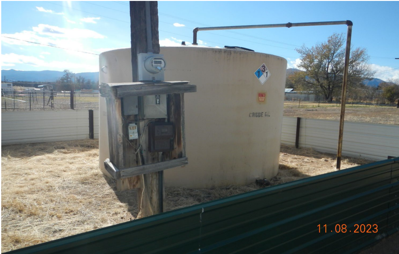
Photo 2. The wires are still exposed on electric breaker box which is a safety issue. Grass was mowed inside the containment but should also be raked up and removed.
