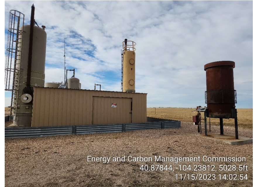
Photo 2 – Heater Treaters and ECD
