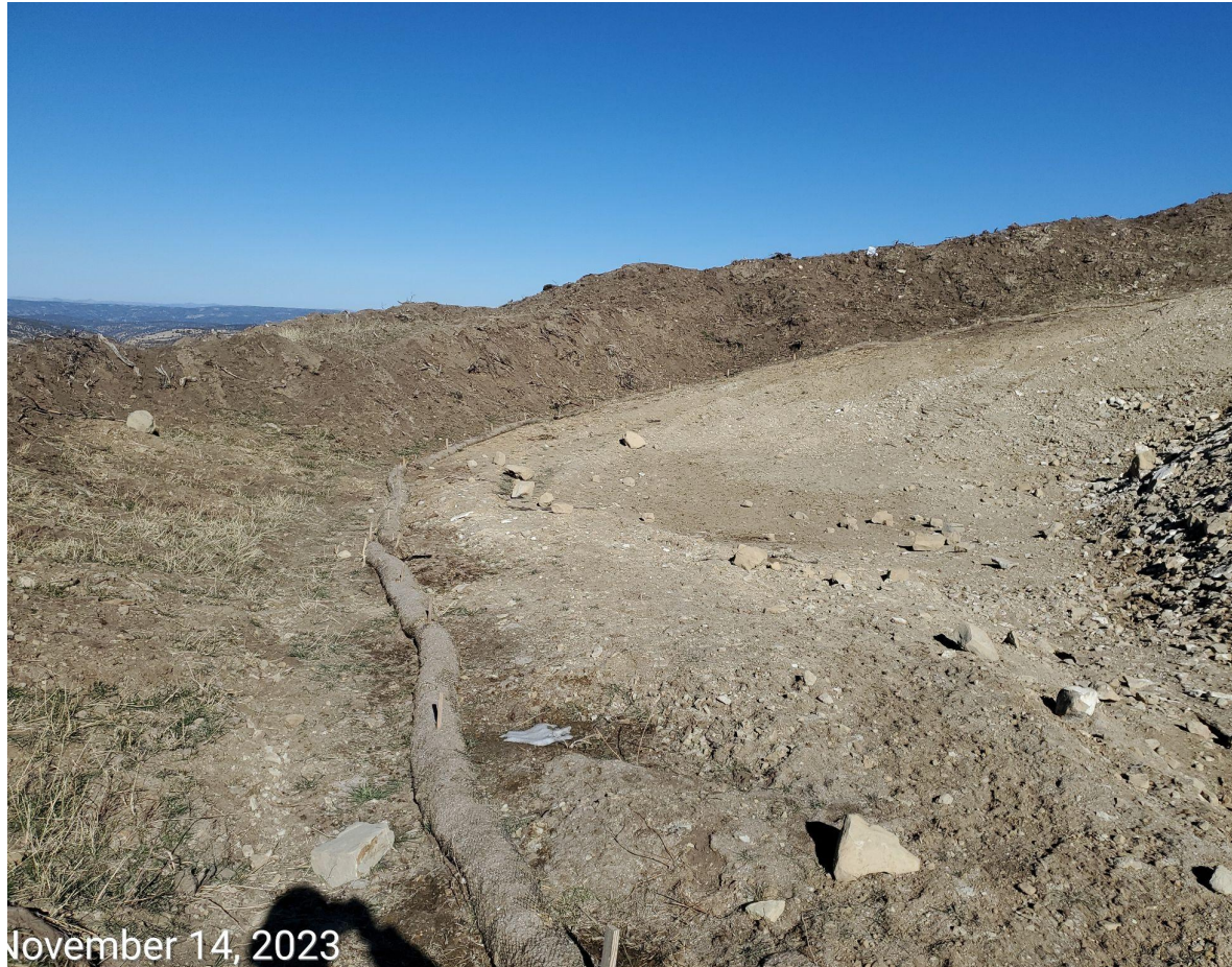
Photo 11: Photo taken from the northwest end of the Location. Photo shows sediment trap #2 appears unchanged in size. Photo also example showing areas of the topsoil stockpiles where hydromulch is no longer in proper functioning condition.
