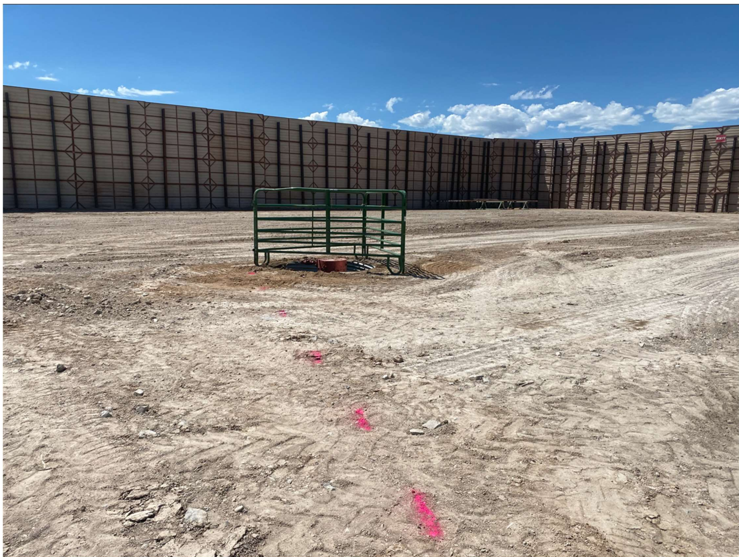
Wellhead and surrounding area. Drill rig and associated equipment was moved off location and the impacted secondary containment liner has been removed and properly disposed of.
