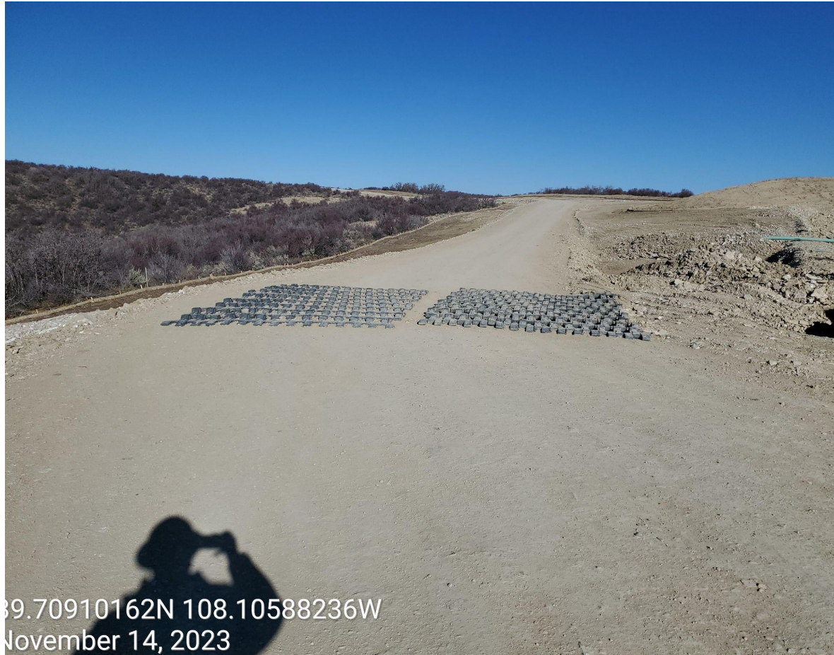
Photo 10: Vehicle tracking pad at the western Location entrance.
