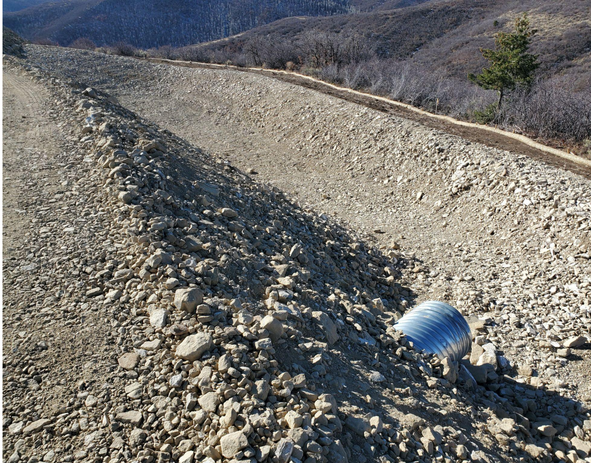
Photo 11: Photo taken from the Location entrance, on the west end of the Location. Photo shows 1 of 3 retention basins constructed on the Location. Retention basin constructed in conjunction with a culvert; basin will only collect stormwater from a small “drainage” along the eastern road (to the secondary access road) on the northwest end of the Location, and not including the working pad surface.
