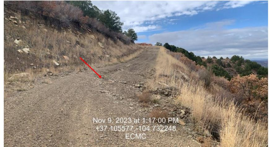
**Photo 7 – Erosion in Roadway**
