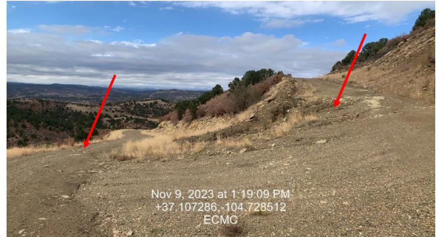
**Photo 5 – Erosion in roadway**
