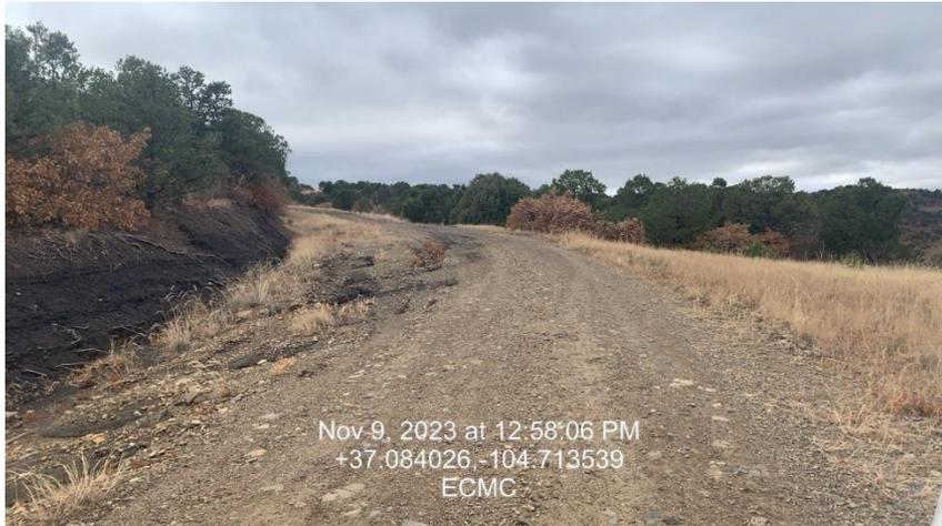
**Photo 9 – Erosion Along Access Road**
