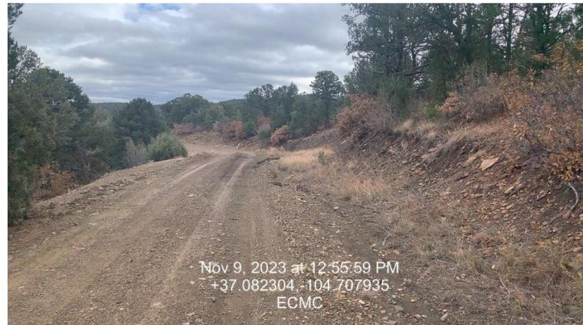
**Photo 7 – Erosion Along Access Road**
