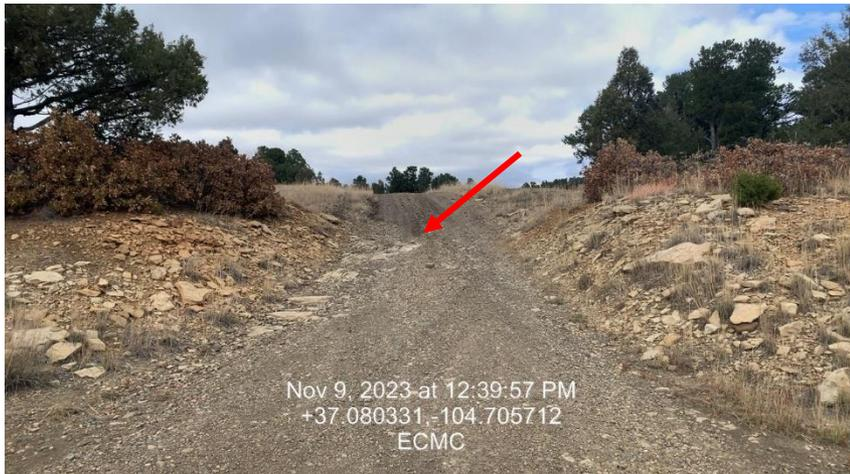
**Photo 5 – Access road with Erosion**
