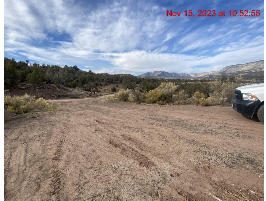
Insufficient Vehicle Tracking BMPs at Location Entrance/Exit – Photo #07558
