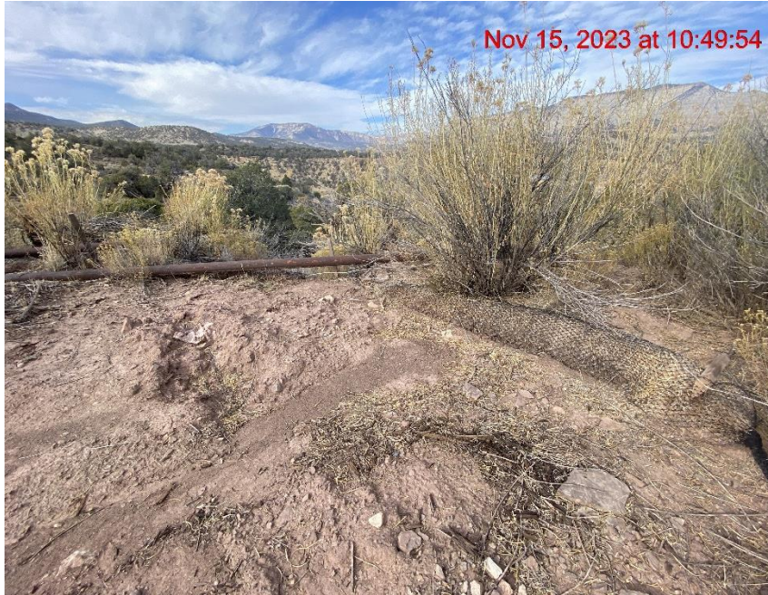
Waddle BMP Degradation— Photo #07554
