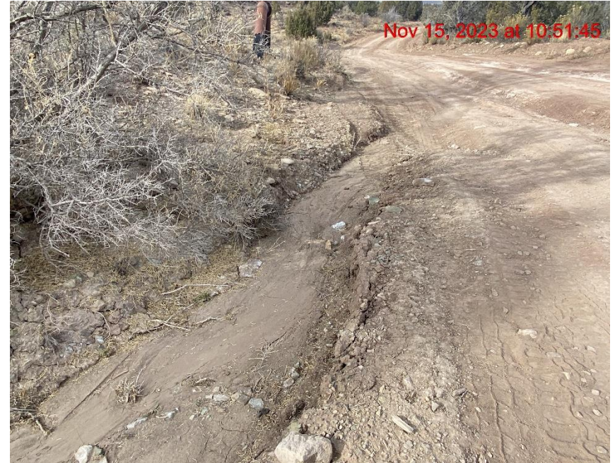
Lease Road Ditch Full of Sediment Running Onto Road – Photo #07556
