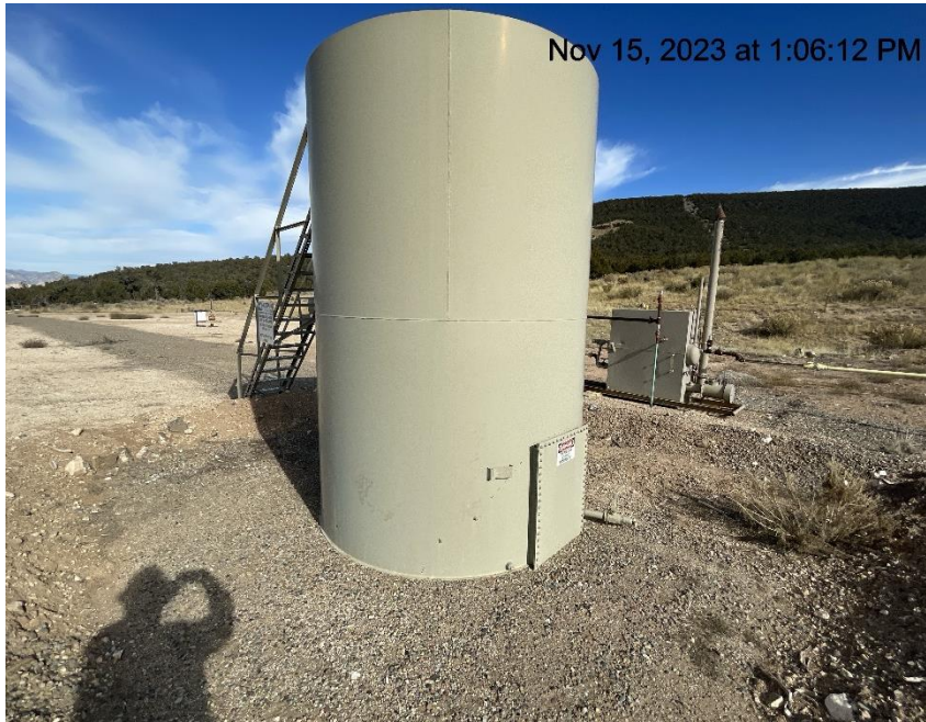
Photo # 6730 Tank not properly labeled/missing required information
