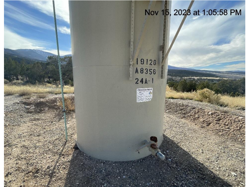
Photo # 6729 Tank not properly labeled/missing required information
