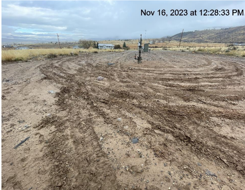
Photo # 6932 Lack of stabilization/compaction/insufficient BMP's
