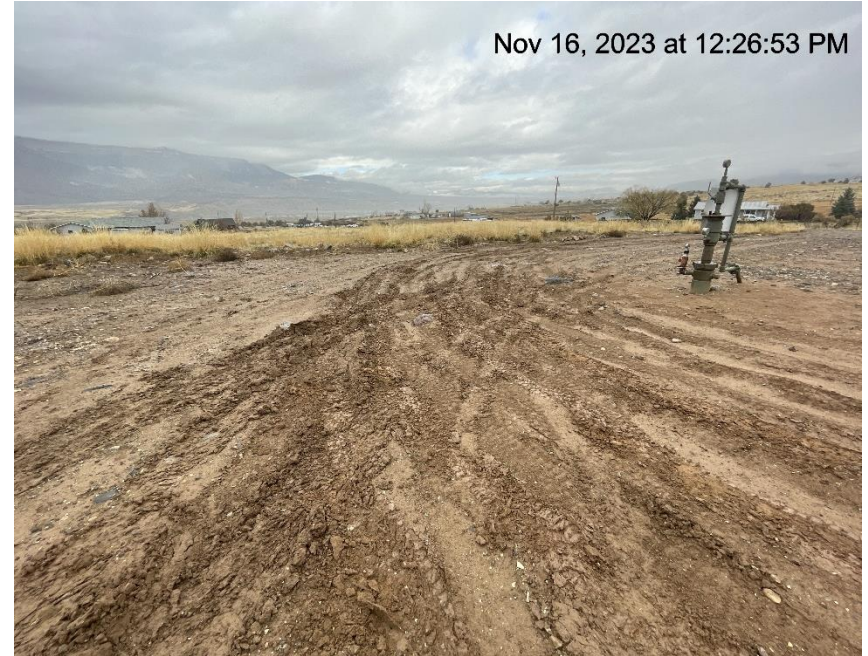
Photo # 6931 Lack of stabilization/compaction/insufficient BMP's
