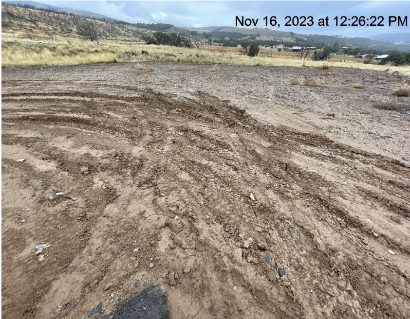
Photo # 6928 Lack of stabilization/compaction/insufficient BMP's
