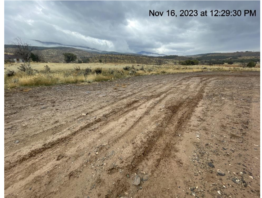
Photo # 6933 Lack of stabilization/compaction/insufficient BMP's
