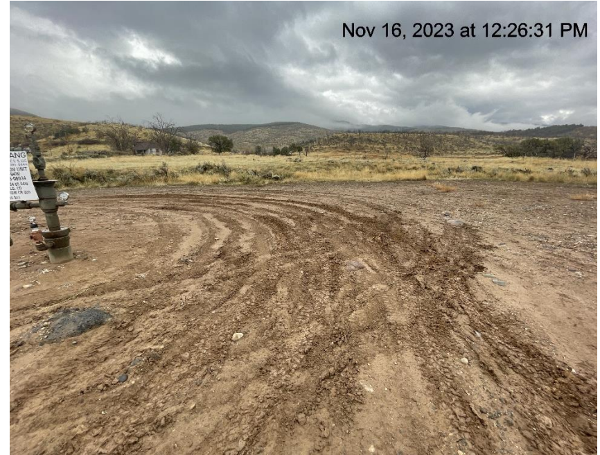
Photo # 6929 Lack of stabilization/compaction/insufficient BMP's
