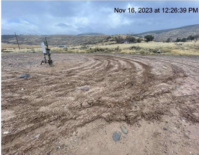
Photo # 6930 Lack of stabilization/compaction/insufficient BMP's
