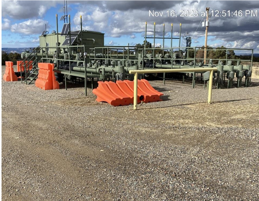
Production manifolds and separator building
