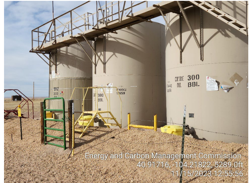
Photo 2 – Tank Battery
