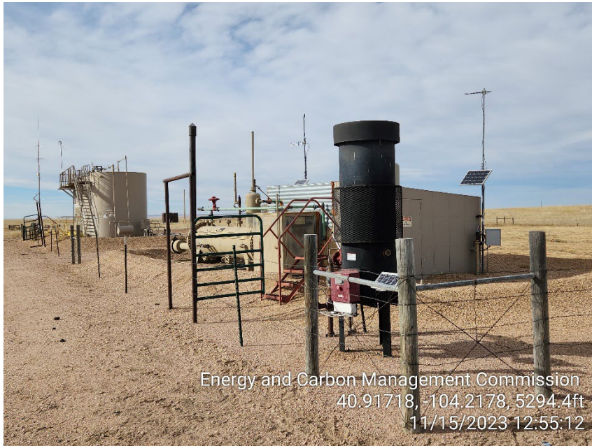
Photo 1 – Separator and ECD
