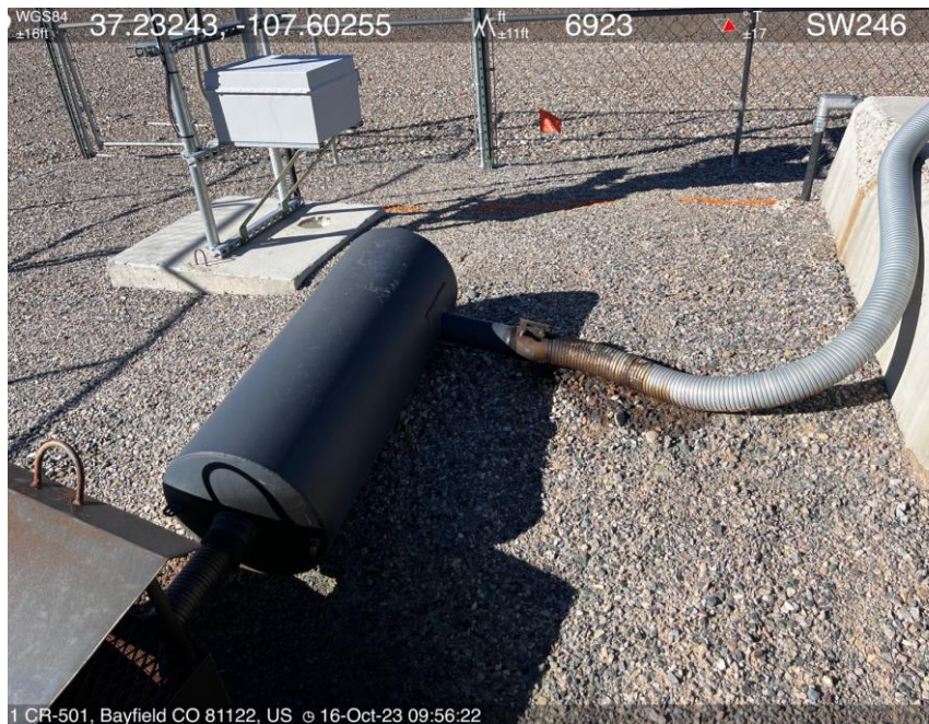
Photo #3. View of corrective action identified in FIR Doc.#712700747.
