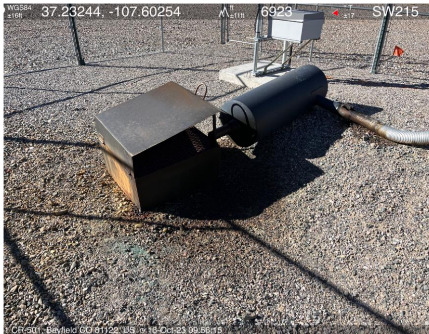
Photo #1. View of corrective action identified in FIR Doc.#712700747.
