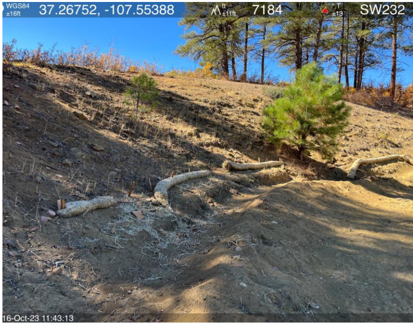
Photo #1. View of corrective action identified in FIR Doc.#712700749.
