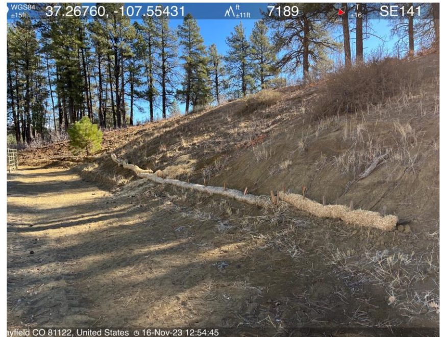
Photo #6. View of completed corrective action.
