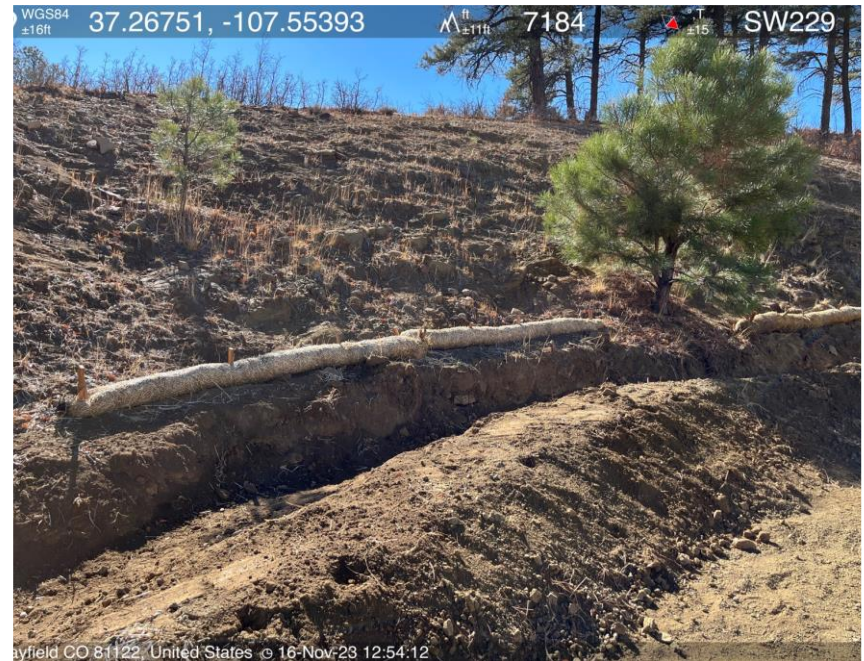
Photo #2. View of completed corrective action.
