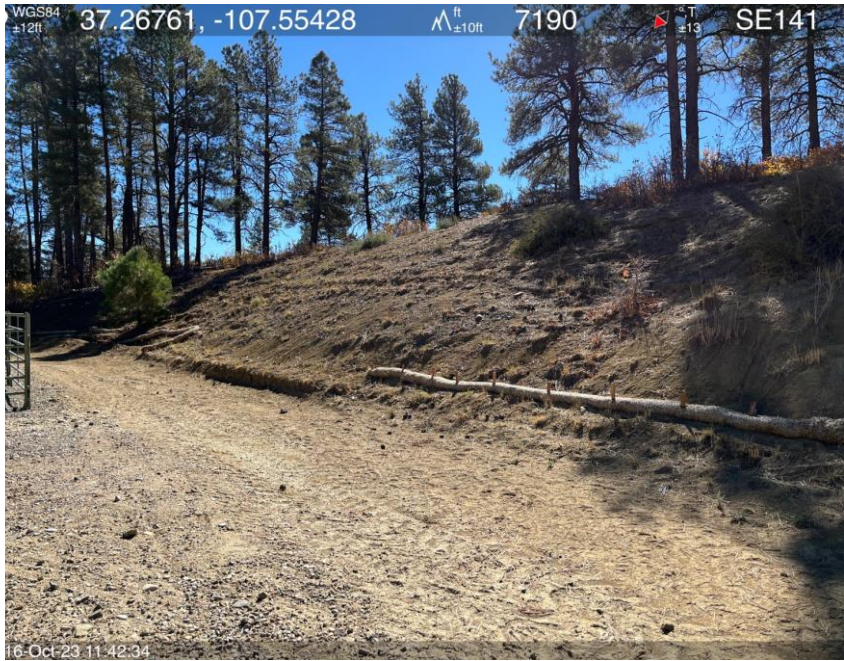
Photo #5. . View of corrective action identified in FIR Doc.#712700749.
