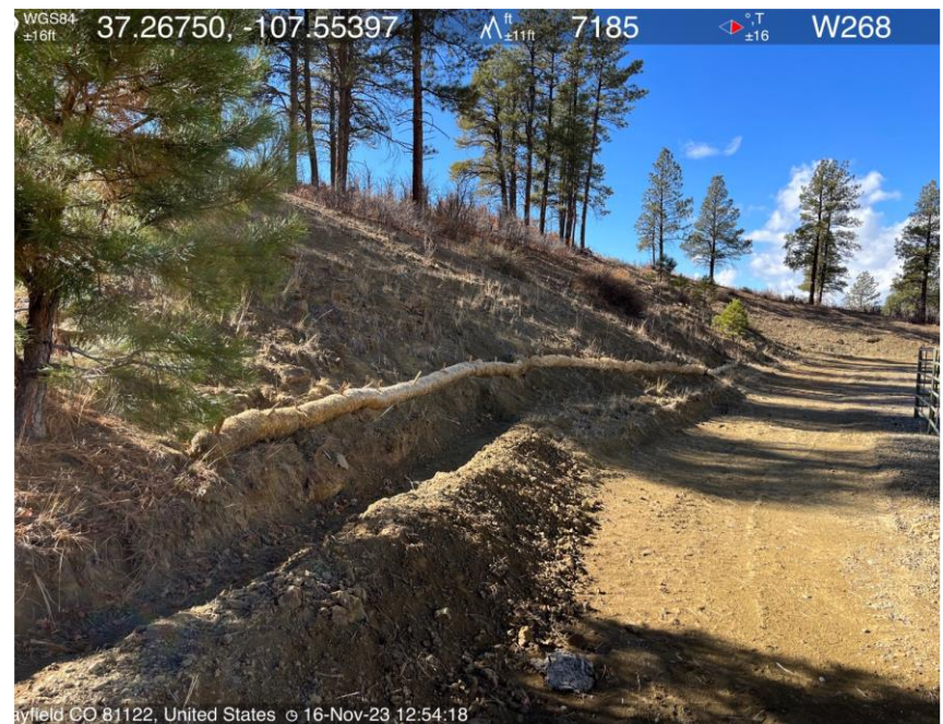
Photo #4. View of completed corrective action.
